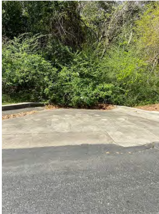
Figure 3-4 Concrete flume that discharges untreated stormwater directly into Carpenter Creek
