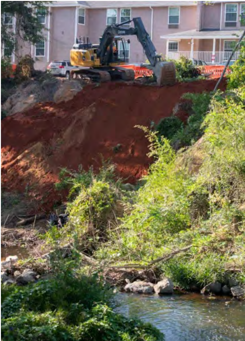
Red clay being used to stabilize an embankment stripped of vegetation near Davis Highway (photo courtesy of the Pensacola News Journal)
