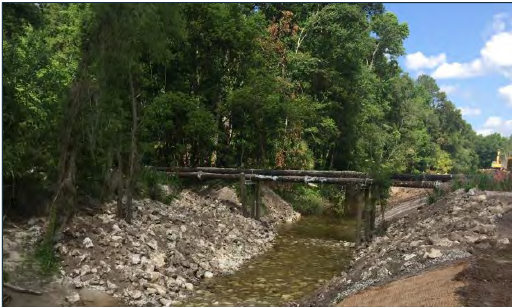
Figure 4.6 – Riprap Channel Protection and Riffle Around Aerial Pipeline
