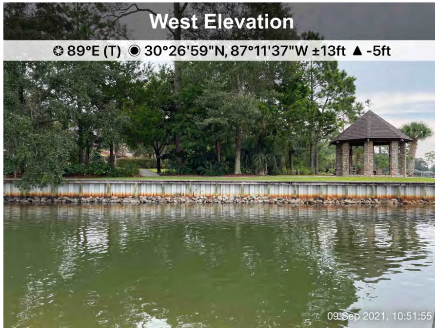
Photograph #33. 2000 Villafane Drive. Large estate home located just southeast of Seville Street outfall. This property is armored by vertical wall faced with quarried limestone. Dense band of submersed aquatic vegetation (wild celery) along the entire waterfront.
