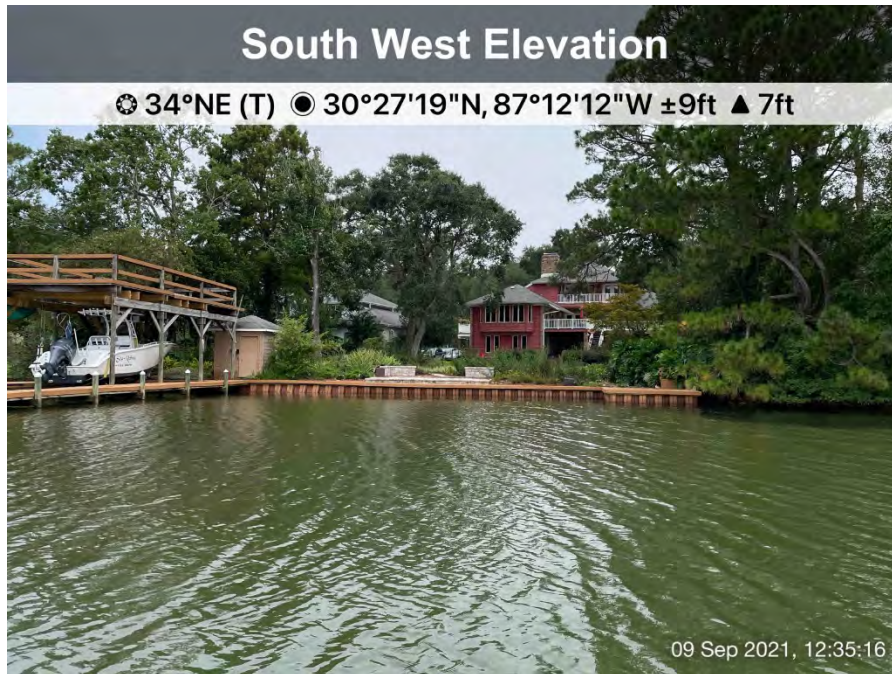
Photograph #53. 681 Tennyson Place. East shoreline of the Bayou. Common example of typical shoreline stabilization method for single family residence along the bayou. Vertical sheet pile wall with no rip rap.
