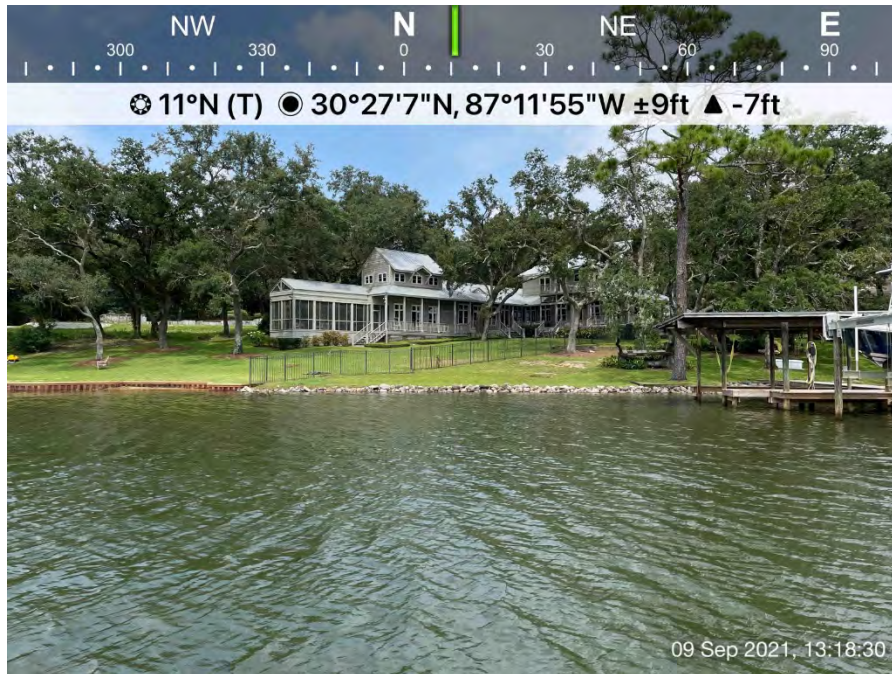
Photograph #61. 371 Woodbine Drive. East shoreline of the Bayou. Two shoreline stabilization techniques including vertical wall with no rip rap (left) and rip rap revetment (right). Submerged lands proximal to the shoreline comprised of submersed aquatic vegetation consisting of wild celery.
