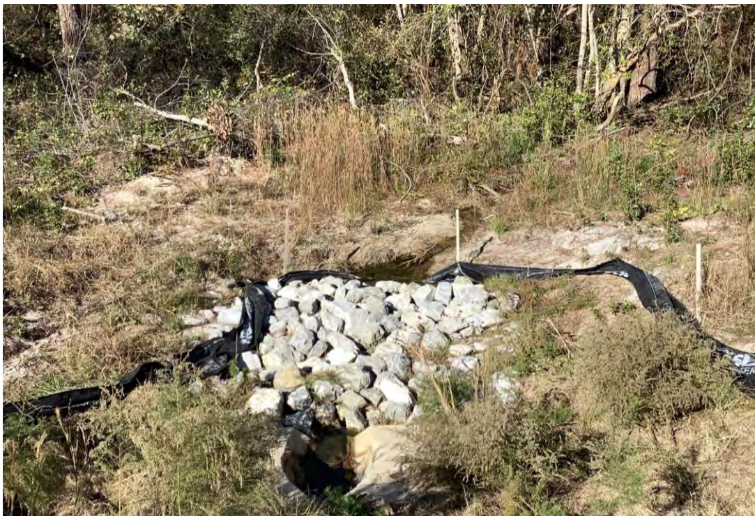
Photograph #8: Site 46 (FPZ 2) Outfall structure into wetland buffer area
