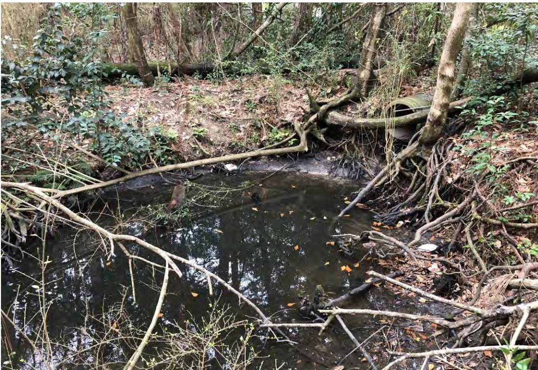
Photograph #70: Site AHI (FPZ 6) Un-armored outlet structure with large blow out
