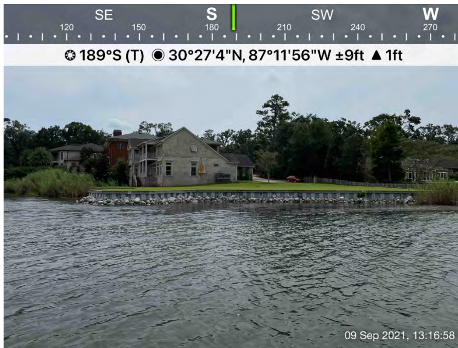
Photograph #60. 3420 North 18 th Ave. Shoreline armored with vertical wall faced with quarried limestone. Broad area of submersed vegetation consisting of wild celery waterward of the existing rip rap to depths of -4-ft.
