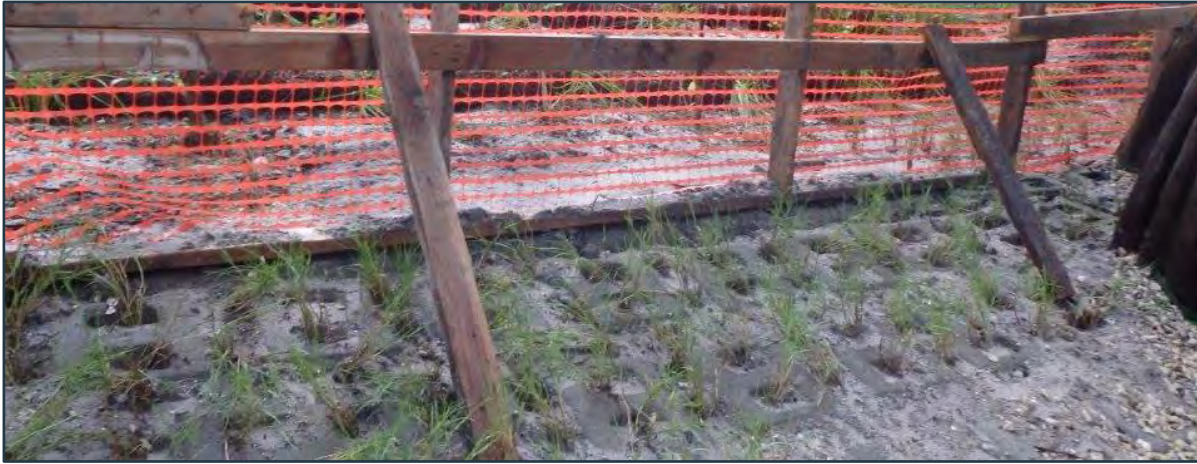
Figure 4.7 – Open Cell Articulated Concrete Block Integrated into a VRSS Foundation
