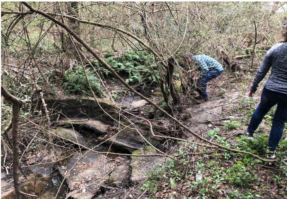
Photograph #72: Site AHI (FPZ 6) Failing concrete outfall
