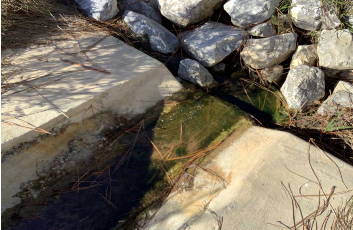
Photograph #9: Site 46 (FPZ 2) Newly constructed outfall structure with algal growth
