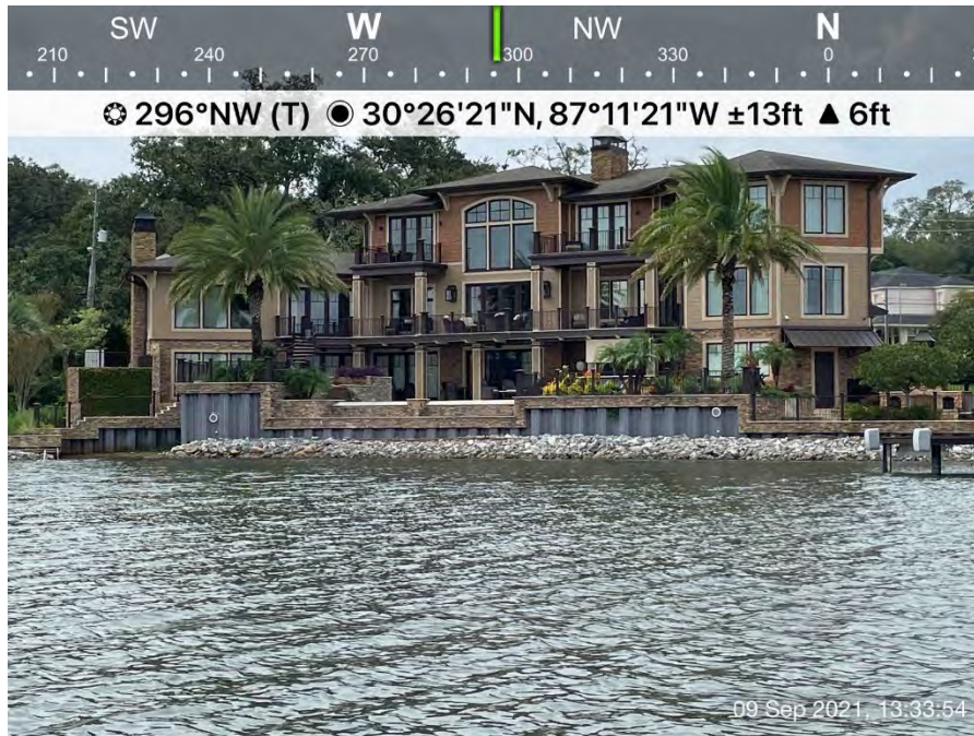
Photograph #67. 2120 Whaley Ave. West shoreline of Bayou. Heavily armored shoreline consisting of stepped vinyl wall with Class II limestone rip rap.
