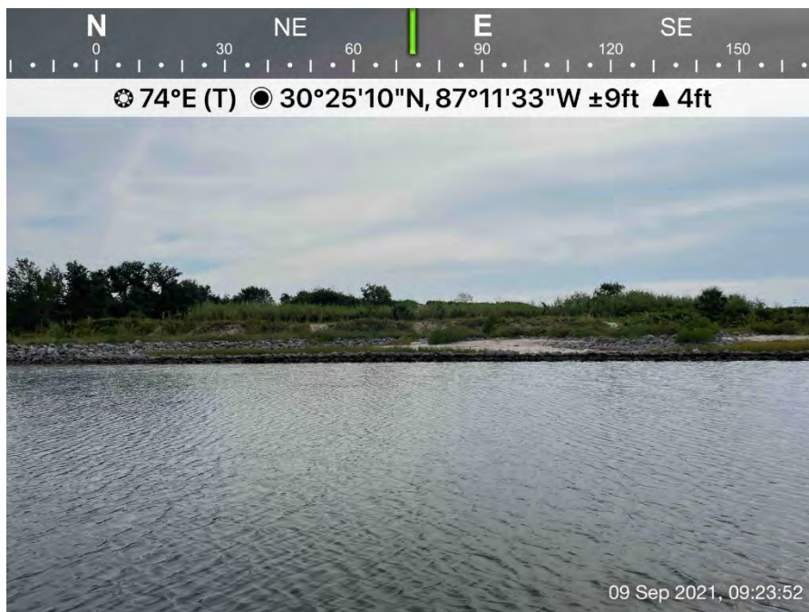
Photograph #6. Condition of east shoreline along the mouth of Bayou Texar just south of the railroad bridge. Shoreline armored with quarried limestone. Upland areas landward of the armored shoreline used as a dredge disposal site so native plant communities are altered.
