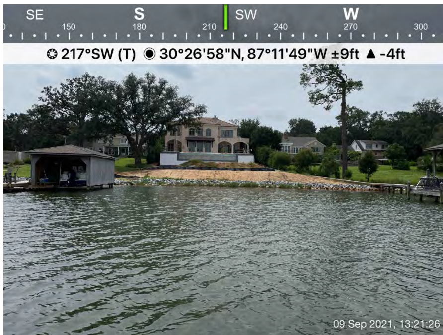
Photograph #62. 3012 Blackshear Ave. West shoreline of Bayou. Example of ineffective BMPs during construction. No barrier in place to keep exposed sediments from eroding into the Bayou.
