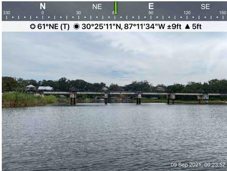
Photograph #7. Railroad bridge that crosses the mouth of Bayou Texar. Structure is supported by steel piles with concrete pile caps.
