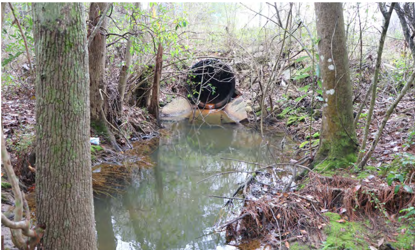
Site Walk Location 05. Stormwater outfall and resulting scour
