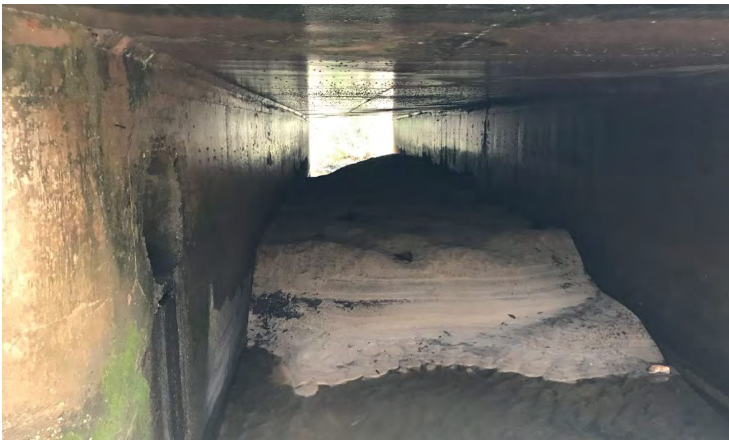
Site Walk Location 20. Sediment trapped under 9th Ave Bridge
