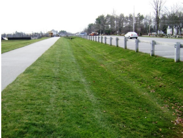
Figure 16 Typical Median Construction to Manage Stormwater Runoff
