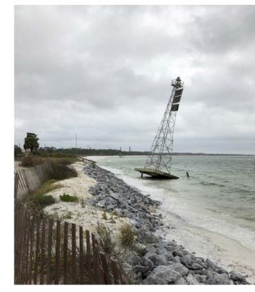
Site C: Looking northeast. Note U.S. Coast Guard Range Tower leaning at eroded shoreline.
