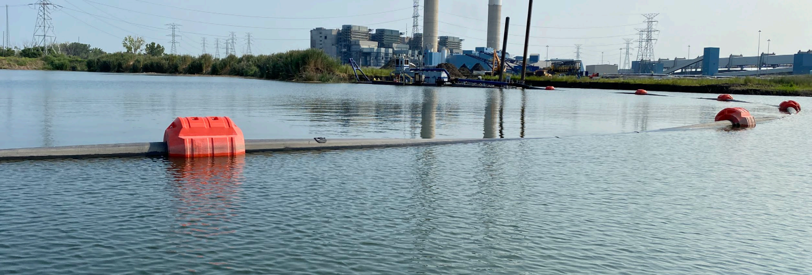
Floating Dredge Discharge Pipe
