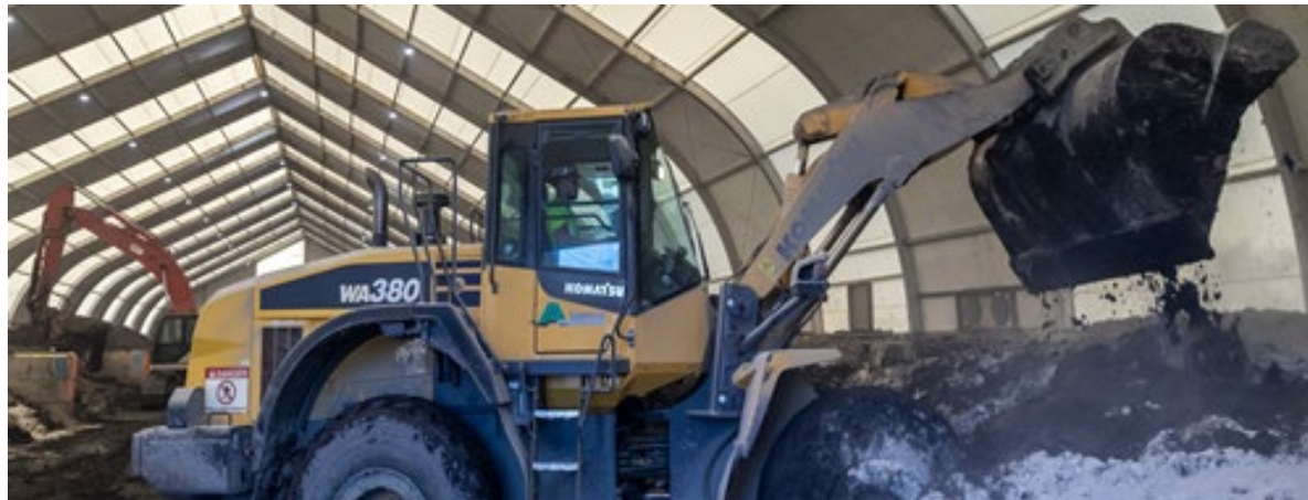
Solidification/Stabilization Reagent Mixing
