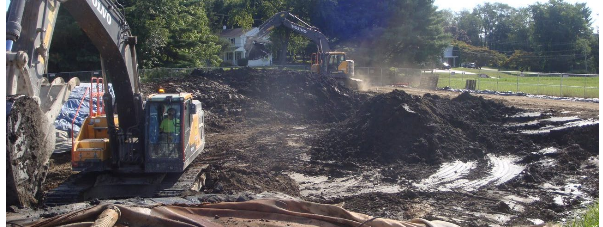
Geotextile Tube Excavation
