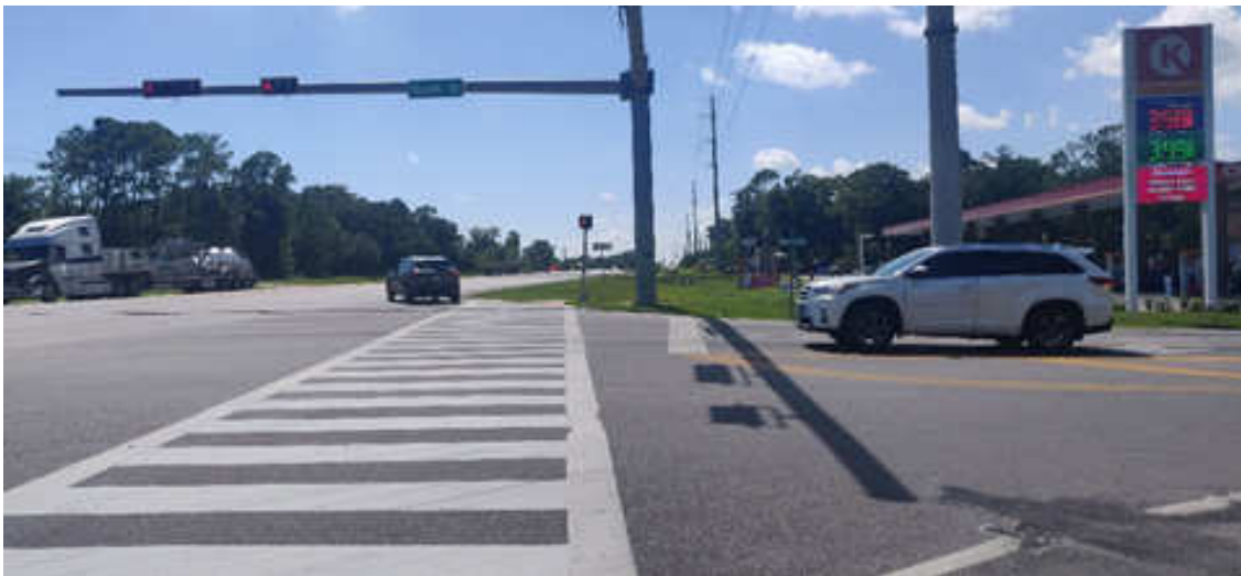
Image: A signalized crossing along Nine Mile Rd (US 90A) with high-visibility crosswalk, detectable warning surfaces, and pedestrian signals.
