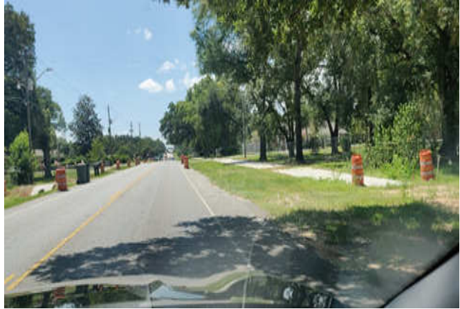
Image: Shared Use Path along Longleaf Dr, still under construction at time of photo.
