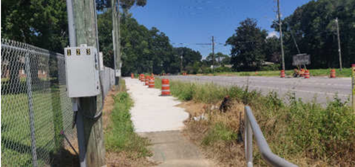
Image: Under construction side path on Longleaf Dr.
