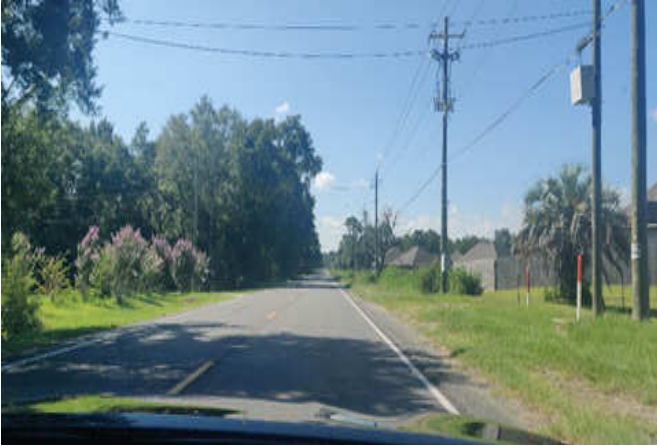
Image: Bikeable paved shoulder along Mobile Hwy (US 90).
