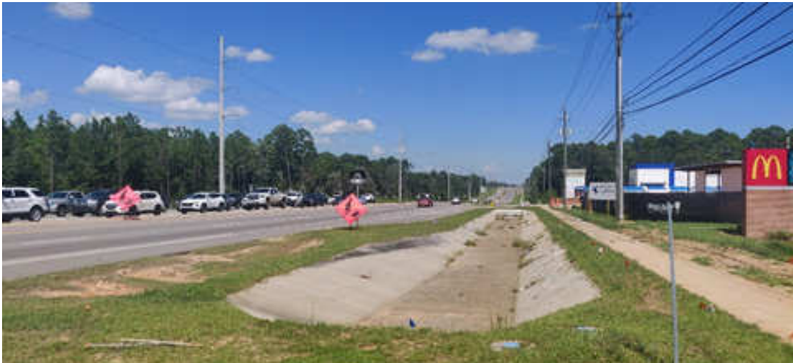
Image: Newly completed sidewalk on the south side of Nine Mile Rd (US 90A)
