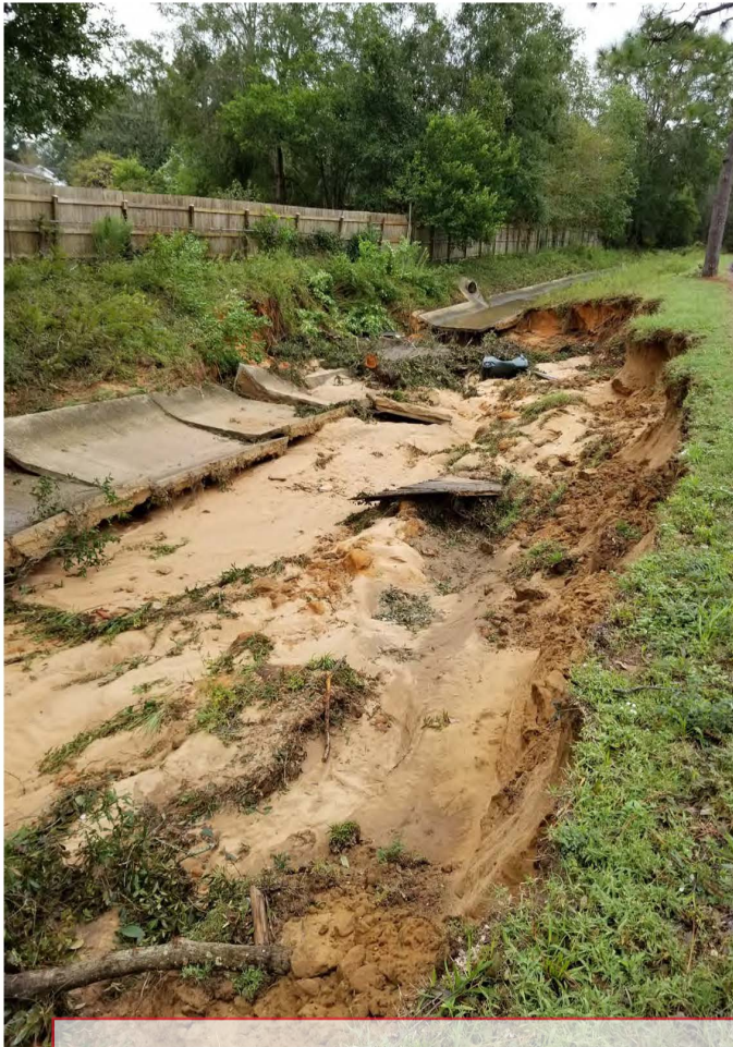
Gatewood Ditch Hurricane Sally Damage (Downgradient from Pond 62)
