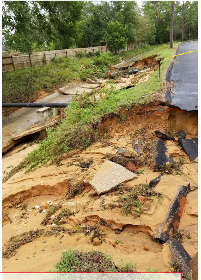
Gatewood Ditch Hurricane Sally Damage (Downgradient from Pond 62)
