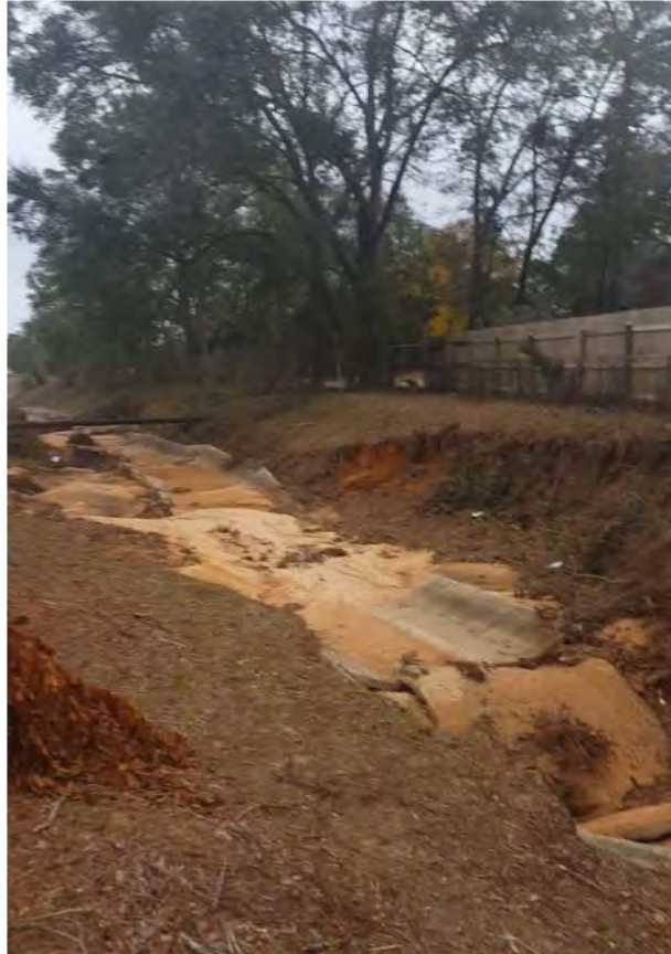
Essex Apartments – Scour, Erosion, and Sedimentation – Expanding – DR#1
