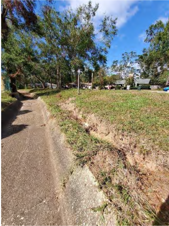
TOD Scour and Ditch Upheaval – 700' West of Tonbridge Drive – Facing West: DA#6
