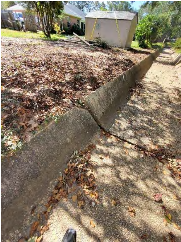
Ditch Upheaval and TOD Scour – 100' West of Tonbridge Drive – Facing West: DA#6
