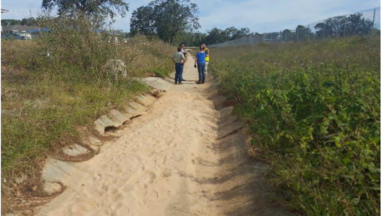
Essex Apartments – Concrete Outfall Ditch: Sedimentation, Concrete Upheaval: DR#2
