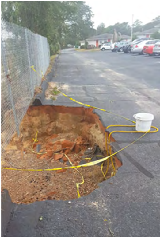
Essex Apartments – Scour, Erosion, and Sedimentation – Expanding – DR#1
