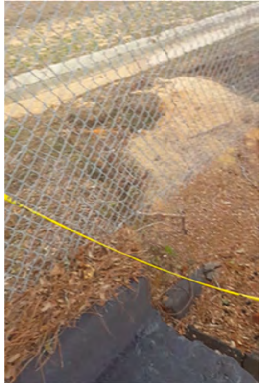
Essex Apartments – Scour, Erosion, and Sedimentation – Expanding – DR#1
