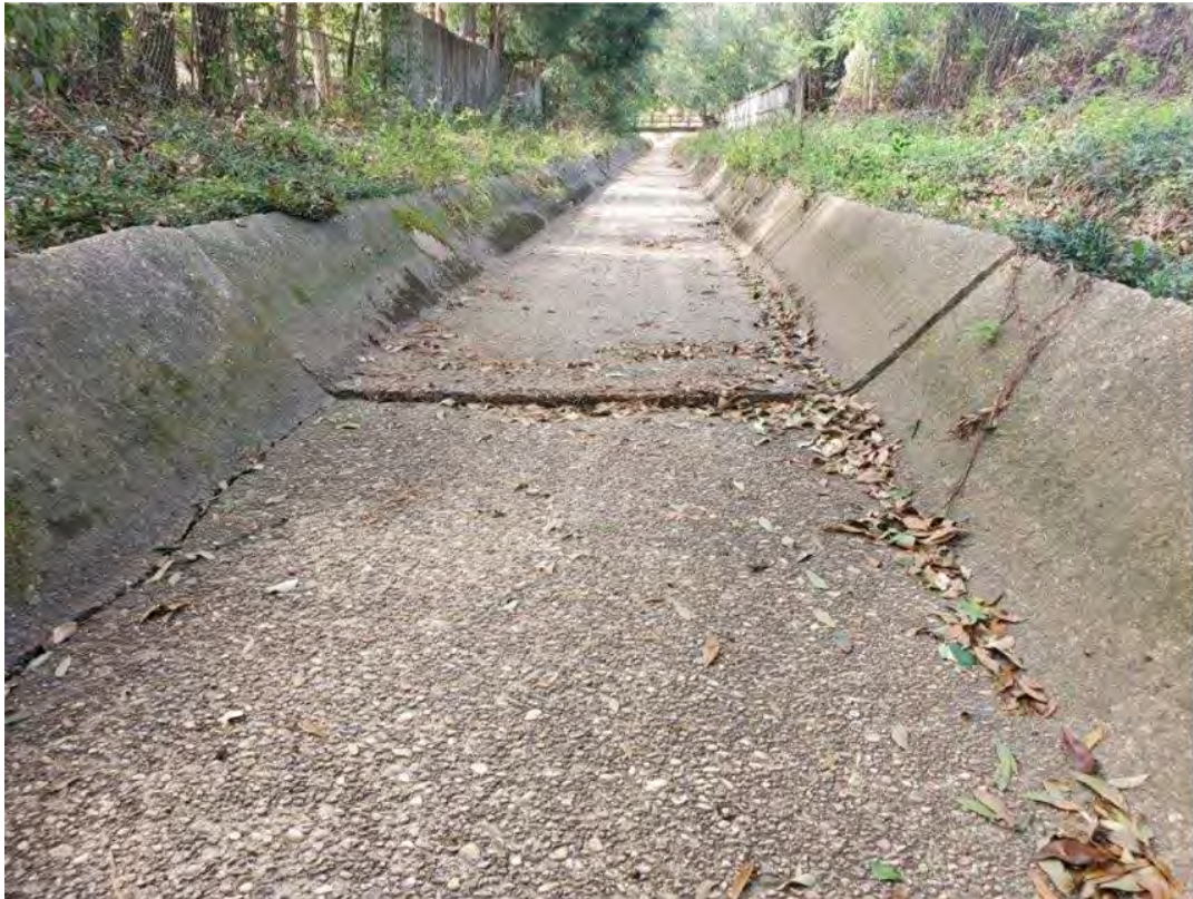
Concrete ditch uplift 100' east of Lyric Lane Bridge – Facing West: DA#5
