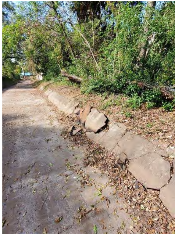
Asphalt Ditch Upheaval/ Failure – 900' West of Tonbridge Drive – Facing West: DA #6
