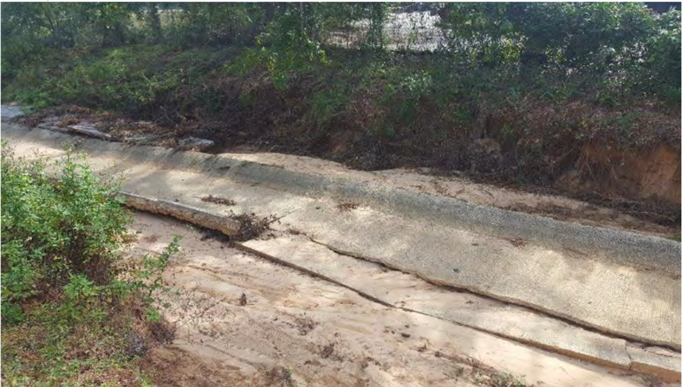
Essex Apartments – Concrete Outfall Ditch: Sedimentation, Concrete Upheaval: DR#3
