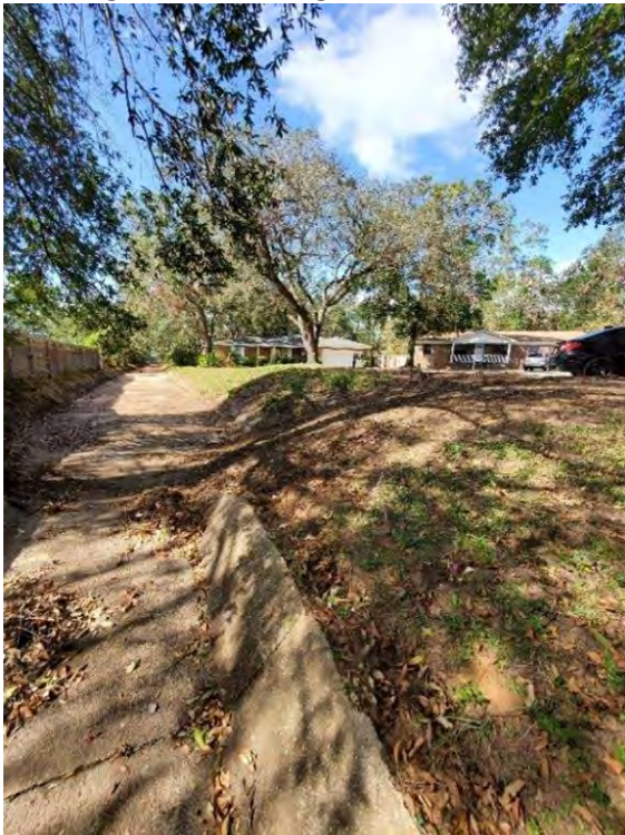
20' to 8' ditch transition – TOD Scour – 800' West of Tonbridge Drive – Facing West: DA#6
