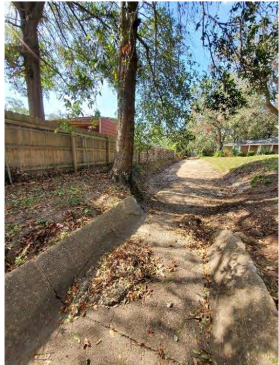
20' to 8' ditch transition – TOD Scour & Ditch Upheaval – 800' West of Tonbridge Drive Facing West: DA#6
