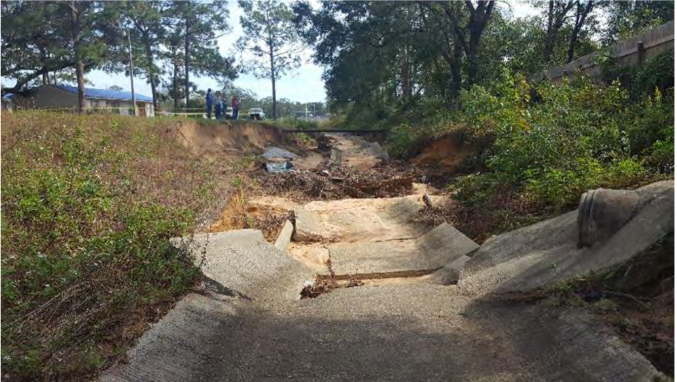
Essex Apartments – Concrete Outfall Ditch - Scour hole, Concrete Upheaval: DR#4
