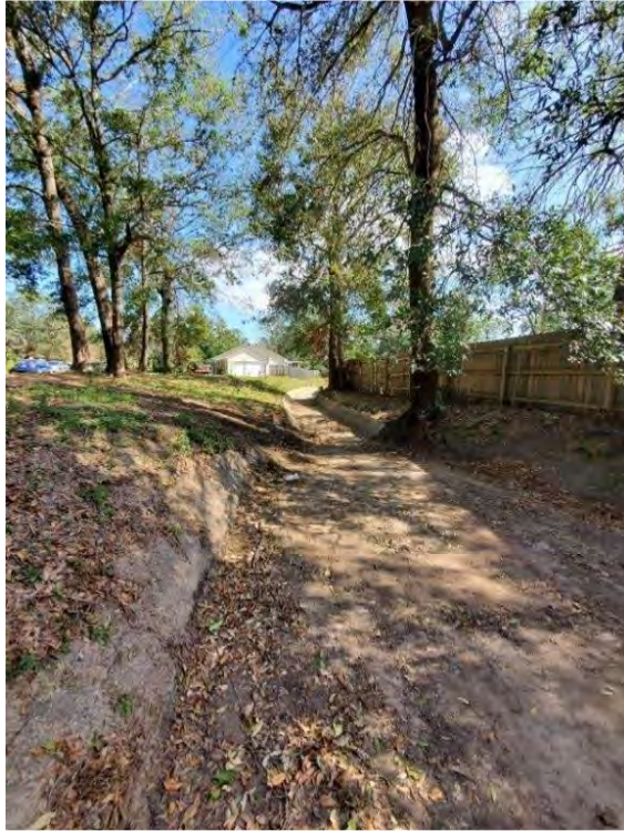
20' to 8' ditch width reduction – TOD Scour & Ditch Upheaval – 800' West of Tonbridge Drive Facing East: DA#6
