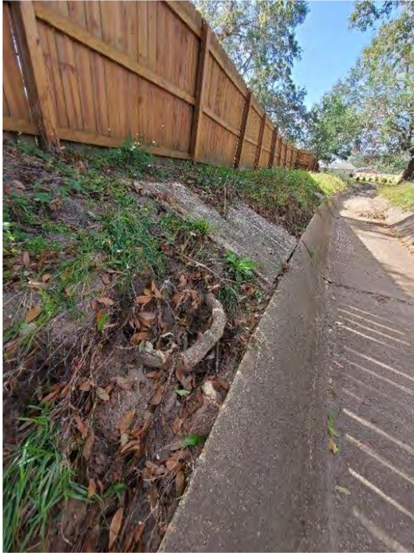
TOD Scour and Ditch Upheaval – 500' West of Tonbridge Drive – Facing West: DA#6
