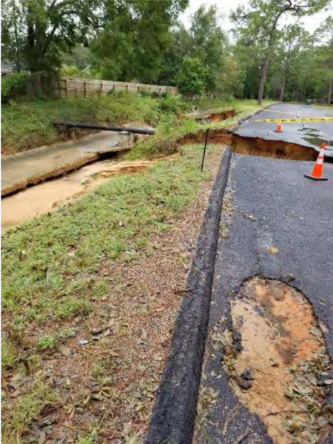
Essex Apartments – Scour hole, Concrete Upheaval: DR#4
