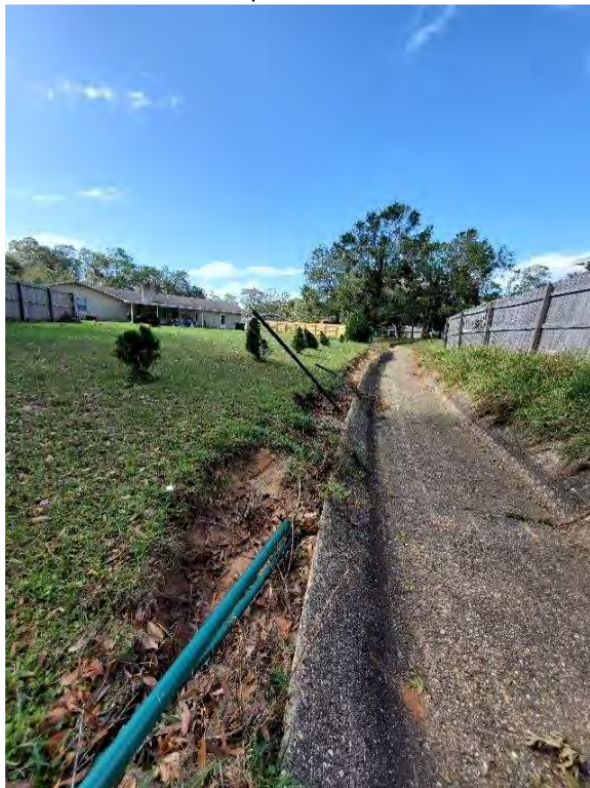
TOD Scour and Ditch Upheaval – 600' West of Tonbridge Drive – Facing West: DA#6
