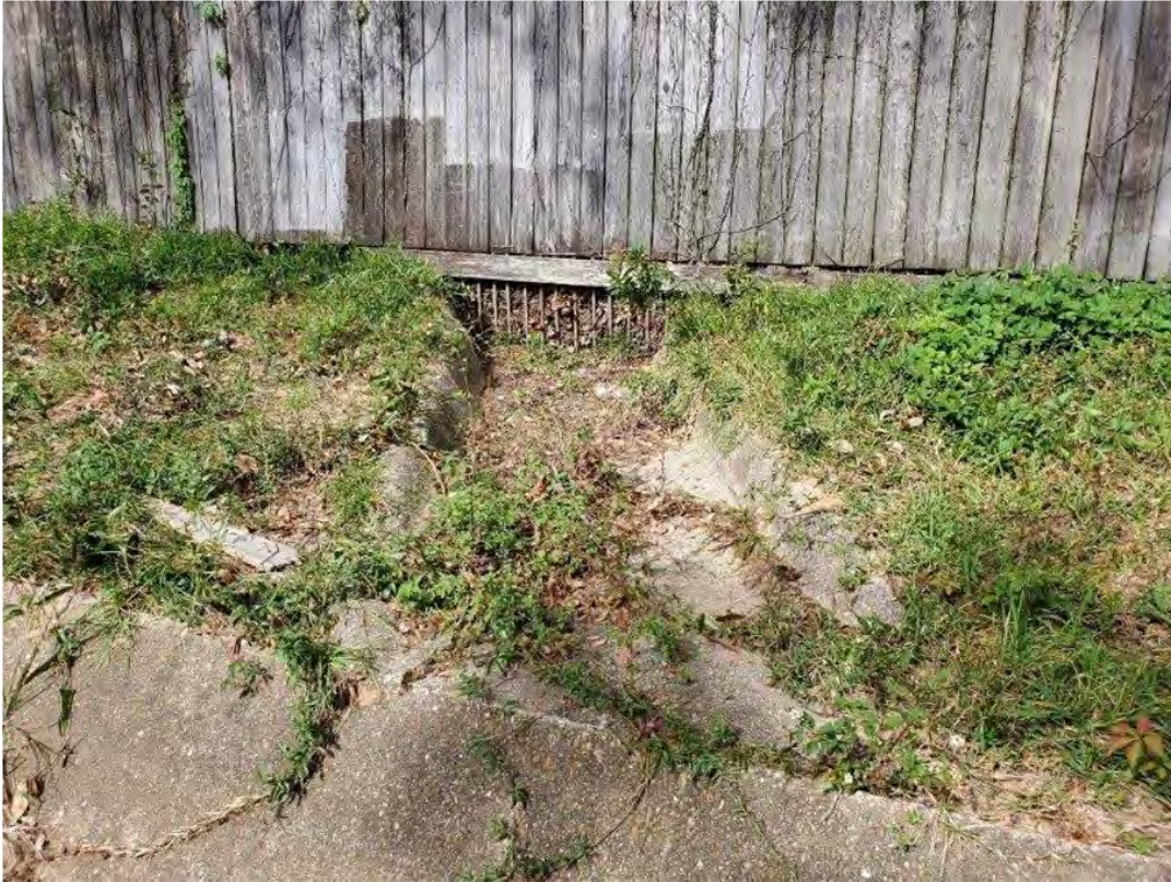
Debris Clogging outfall flume under fence – East Side – Facing North: DA#5
