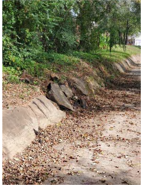
Asphalt Ditch Upheaval/ Failure – 900' West of Tonbridge Drive – Facing West: DA#6
