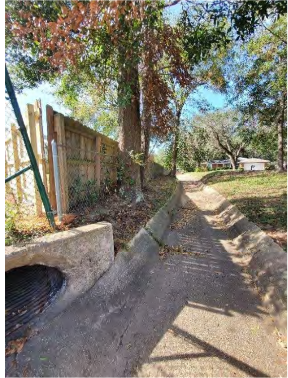
TOD Scour and Ditch Upheaval – 750' West of Tonbridge Drive – Facing West: DA#6
