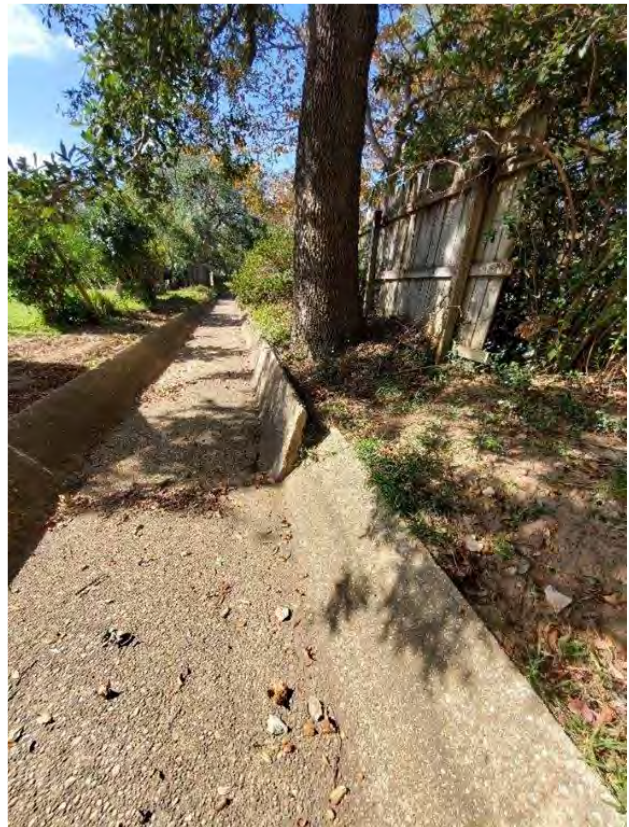
Ditch Upheaval and TOD Scour – 100' West of Tonbridge Drive – Facing West: DA#6
