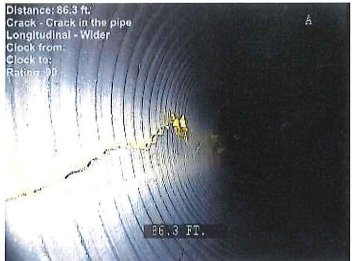
A couple instances of cracks in the pipe between E-104 and E-105. This is one of 25 locations in this run.
