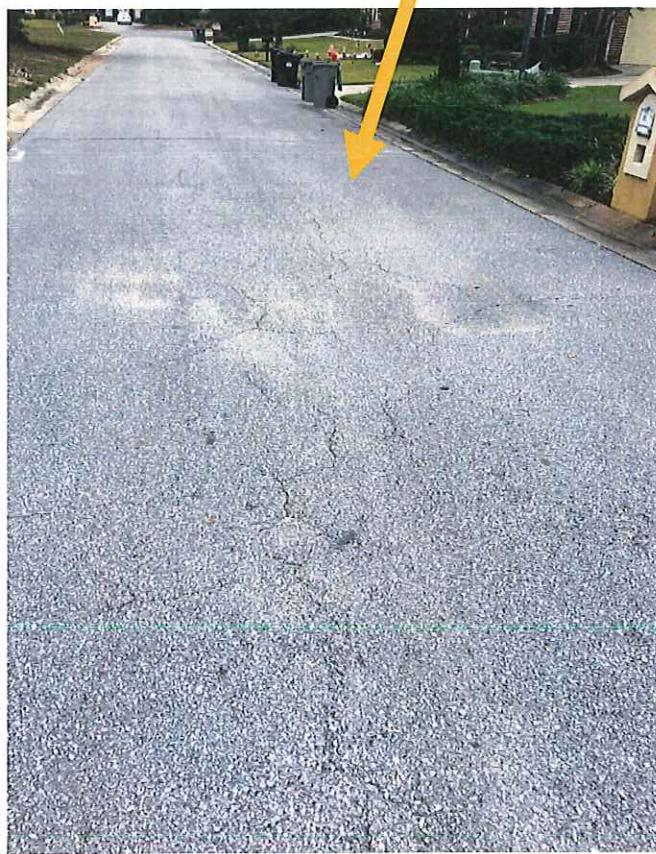
Cracking evident in the pavement between E-103 and E-104.
