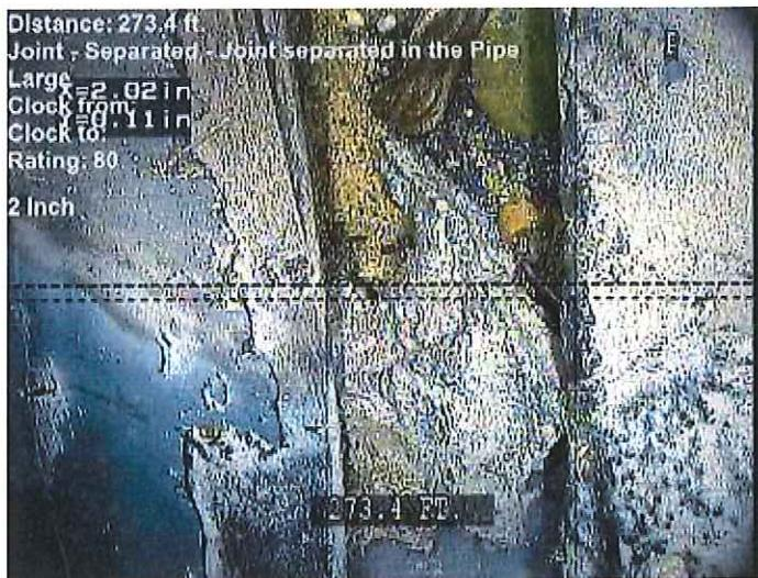
This is a joint separation in the pipe run between E-104 to E-105 near the existing manhole
