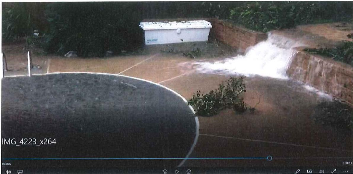
Above is a screenshot of a video taken by the resident of 4525 Baywalk Circle. Flow is coming from the right and flowing to the left to Escambia Bay. The high flows combined with elevation change can cause severe erosion if the earth is not protected. Some evidence of erosion is shown below.
