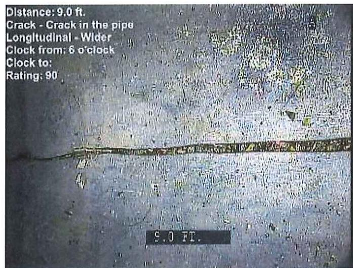
Crack in the polyethylene pipe between E-103 and E-104 in two locations.
