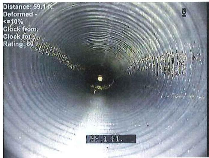
Pipe deformation between E-105 and E-107.
