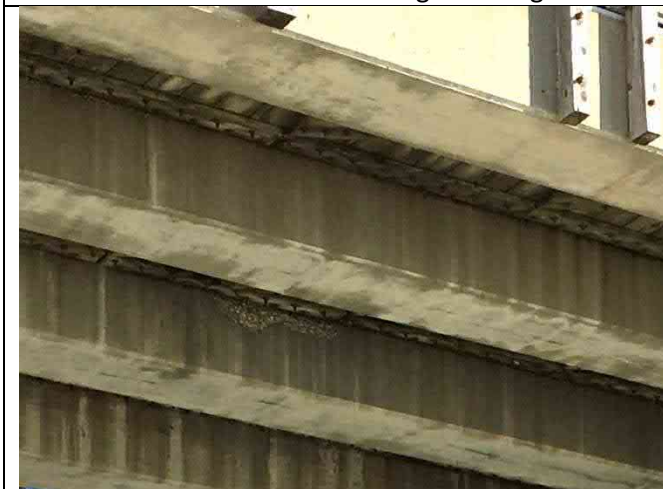
Beam 16-2 – Top flange spall 30"x8"x3"
