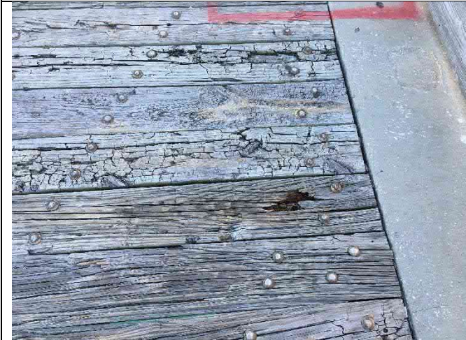
Span 24 – Deck decay
