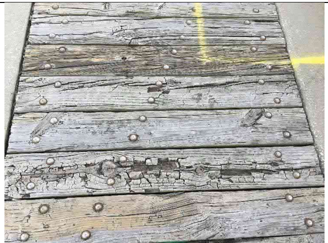
Span 39 – Deck damage with gaps and dips > 0.5"
