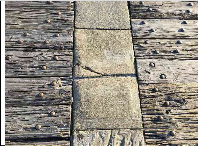
Bent 9 – Closure cracking
