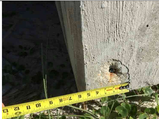
Bent 4W – Pile cap spall 3"x3"x2"
