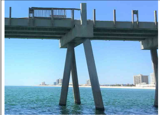
Bent 37E – Previous pile spall repairs in place
