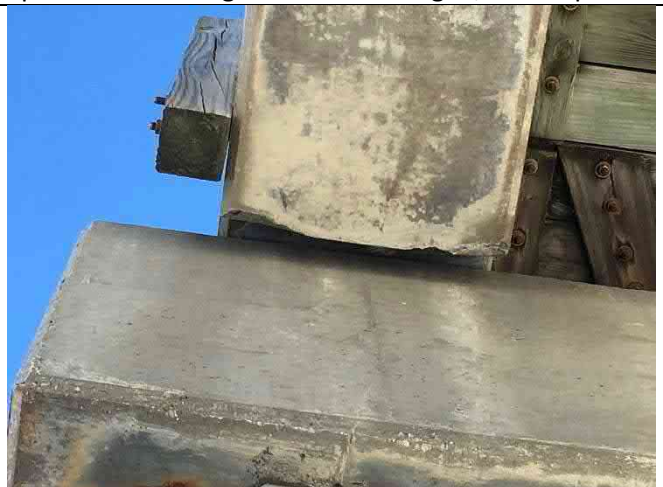
Beam 10-1 South – End spall 24"x3"x3", pile cap hairline crack
