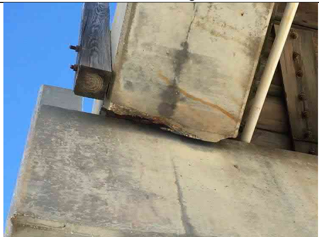
Beam 7-1 South – End cracking and spall 24"x4"x3", longitudinal cracking
