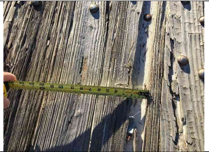
Span 5 - Damaged deck
