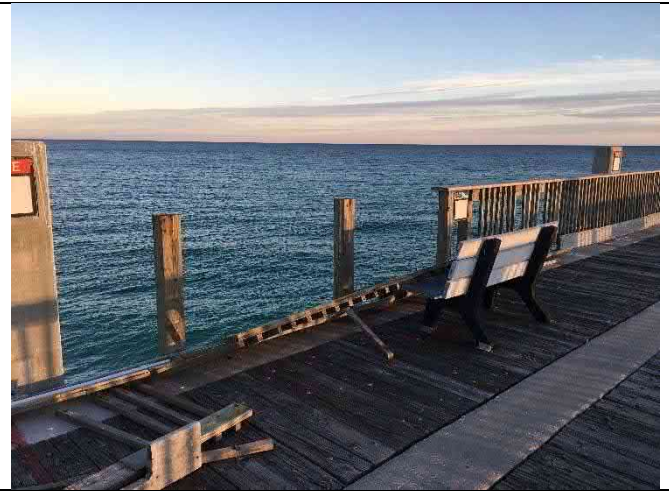
Span 23E – Railing damage
