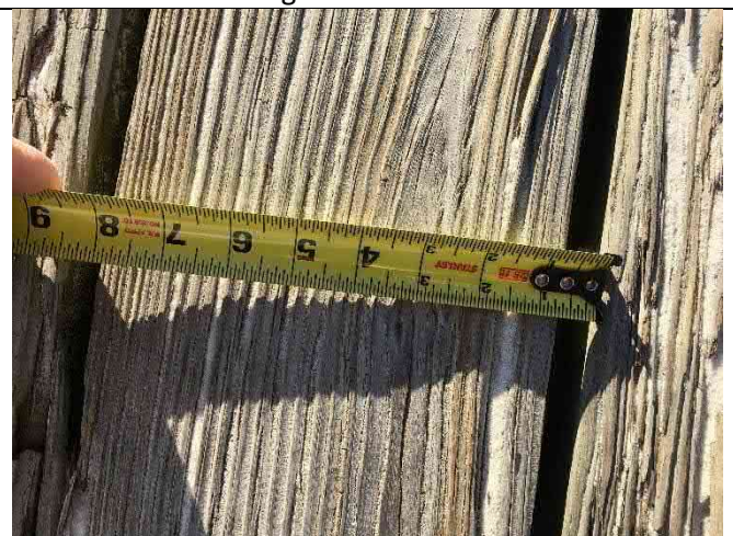
Span 4 – Deck opening greater than 0.5" exceeding ADA 4.5.4 limits.
