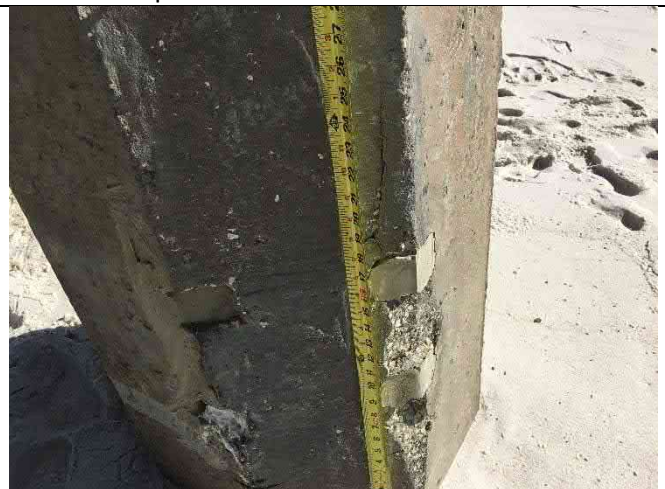
Pile 14-3 – Spall 26"x6"x2", 20"x6"x2"
