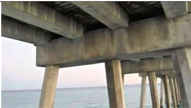
Bent 21 North Face – Beam end cracking
