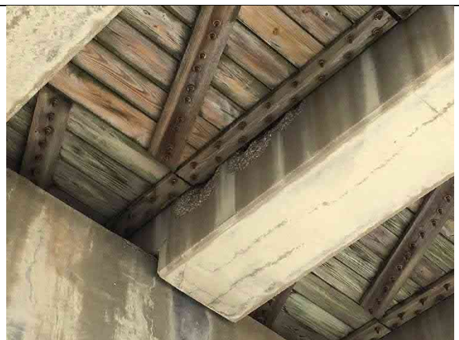
Beam 11-3 South – Top flange spalls 48”x12”x2”, beam end cracking, longitudinal cracking
