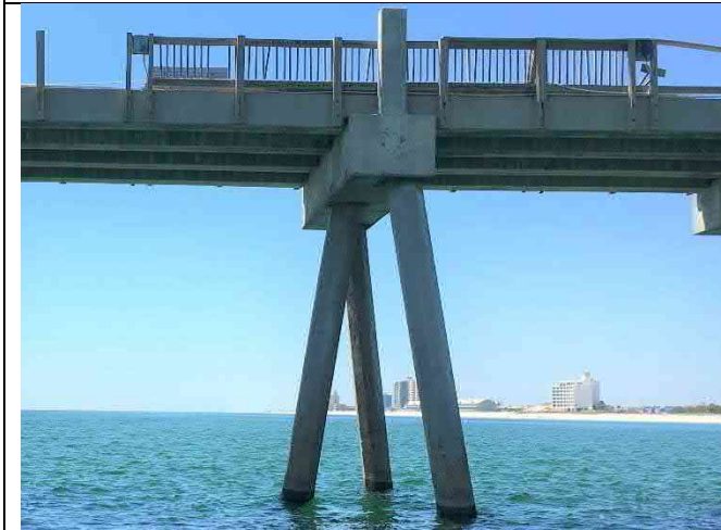
Bent 39E – Pile spall repairs in place but not filling holes 3x4~4"x4"x1"
