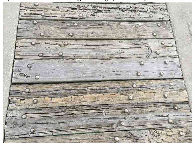
Span 40 – Deck damage with gaps and dips > 0.5"
