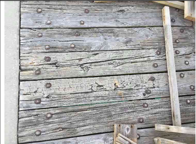
Span 35 – Deck damage with gaps and dips > 0.5"
