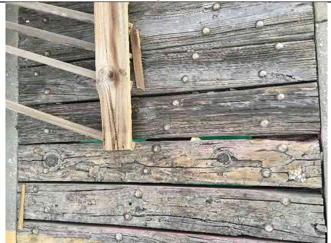
Span 43 – Deck damage with gaps and dips > 0.5"
