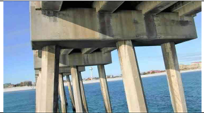
Bent 44 South Face – Beam 44-2 north end cracking, delamination, spall 24"x6"x3", longitudinal cracking
