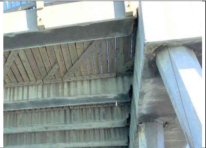
Bent 48W – Beams 48-3, 48-4, 48-5, 48-6 south end cracking, delamination, and spalls 4x24"x12"x3", Pile cap spall around Pile 48-5 30"x30"x4"
