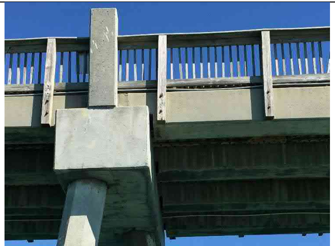
Bent 34W – Beam 34-3 end cracking and delamination
