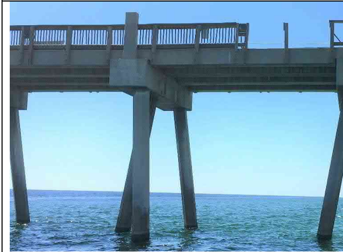
Bent 44E – Pile 44-2 top spall 20"x2"x1", Pile spall repair damage 3x4~4"x4"x1"
