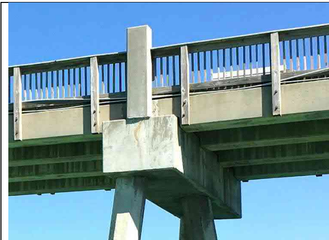
Bent 24W – Span 24 beams shifted north, rust staining under light column, closure pour cracking
