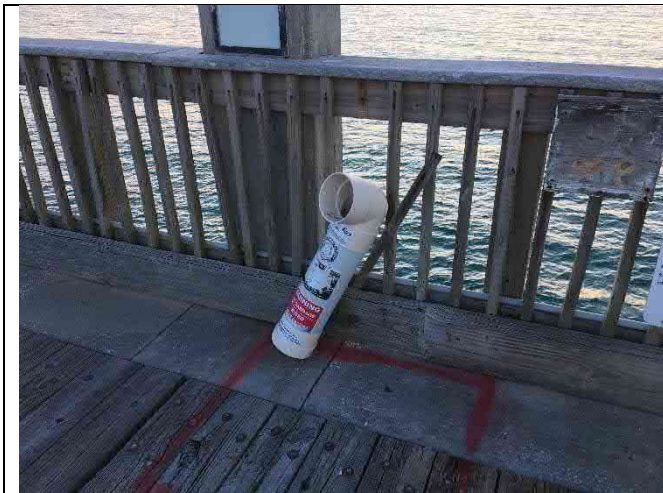
Span 28W at Bent 29W – Fishing line receptacle damage
