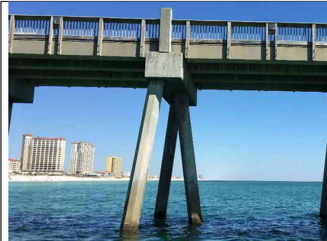
Bent 28W -Beams shifted north
