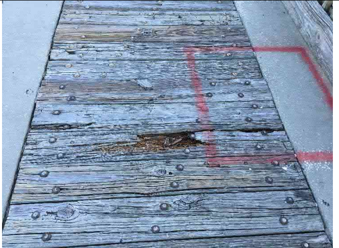
Span 26 – Damaged deck with gaps and dips > 0.5"
