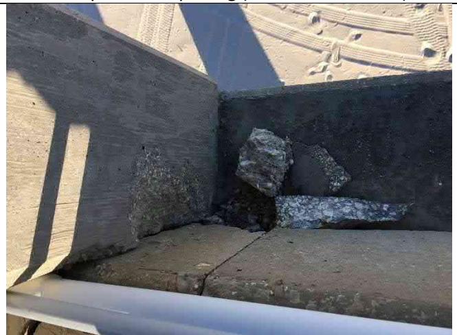
Bent 8E – Light column spall 12"x8"x2", closure spall 12"x6"x4"
