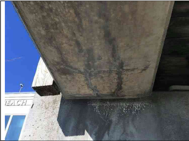
Beam 4-4 North – Bottom flange cracking, spall forming, longitudinal cracking
