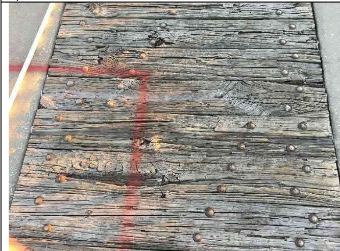
Span 34 – Deck damage with gaps and dips > 0.5"
