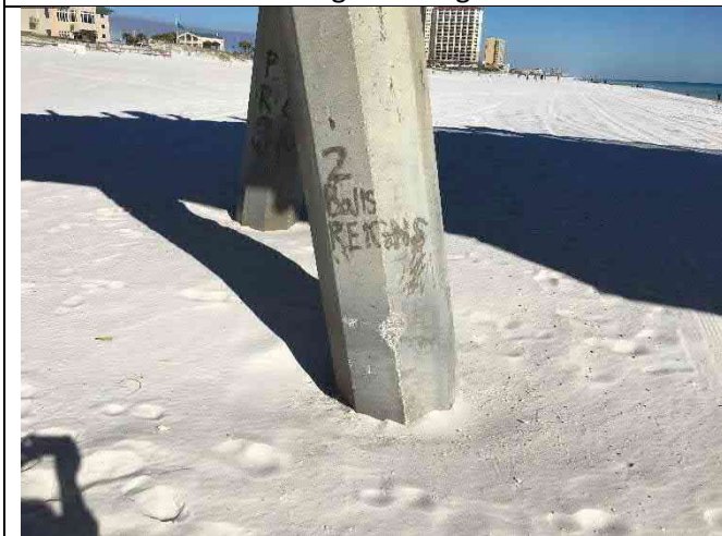
Pile 11-2 – Spall 5"x7"x2"
