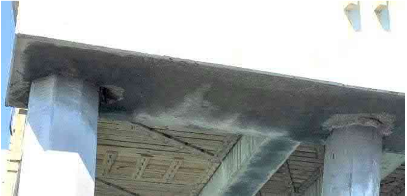
Figure 16 – Pile Cap Spalls around Piles from Lateral Loading
