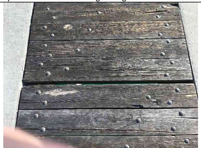
Span 47 – Deck damage with gaps and dips > 0.5"
