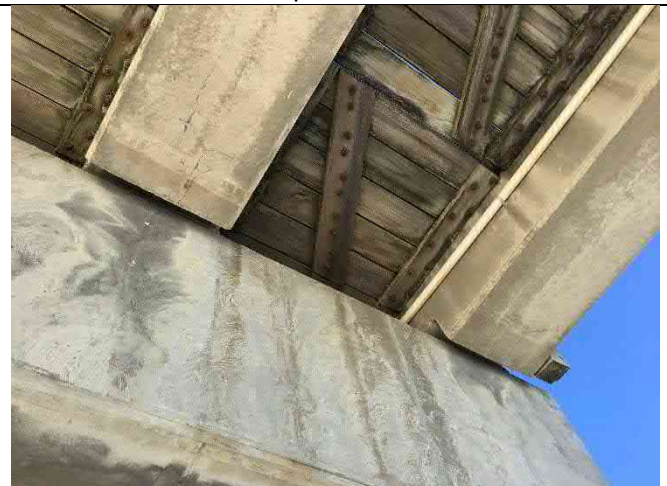
Beams 6-2 and 6-2 North – End cracking and delamination, longitudinal cracking
