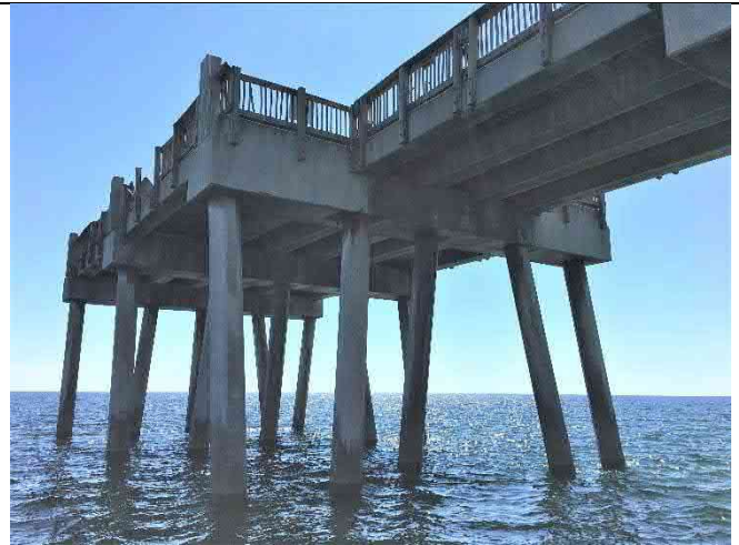
Bent 46E North Face – Pile 46-2 top spall 6"x6"x1"
