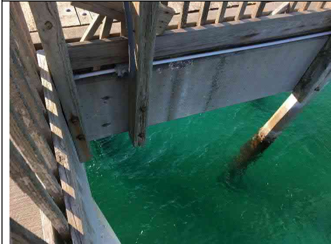
Bent 46E – Beam 45-1 spalls 2~3"x3"x2", spall 12"x3"x2" top flange
