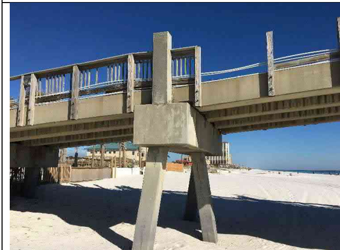
Bent 6W – Split railing post (common condition)
