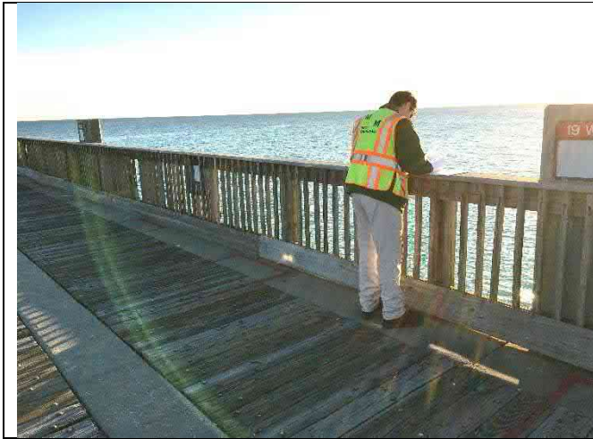
Span 19W – Loose rail with split wood members
