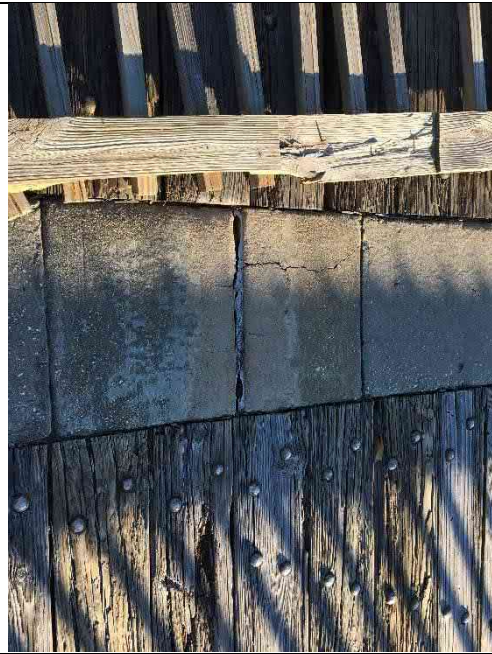
Bent 8 Beam 2 – Closure cracking
