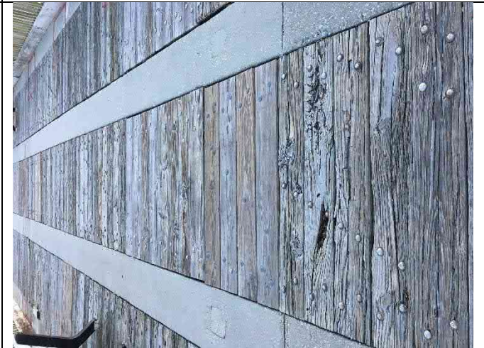
Span 25 Center – Deck damage > 0.5"
