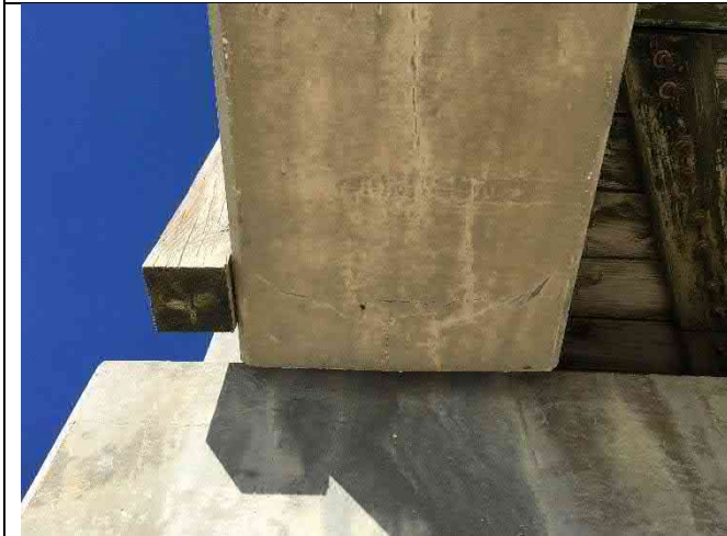
Beam 5-4 North – End cracking and delamination 24"x12"
