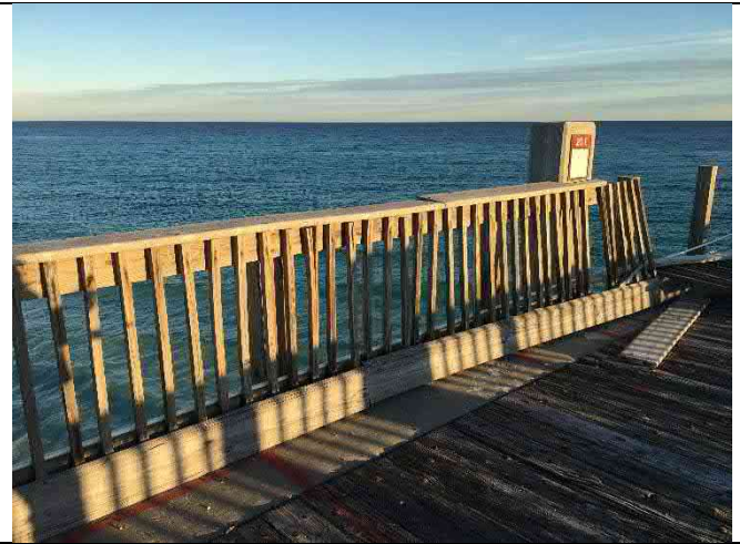
Span 19E – Loose rail with split wood members
