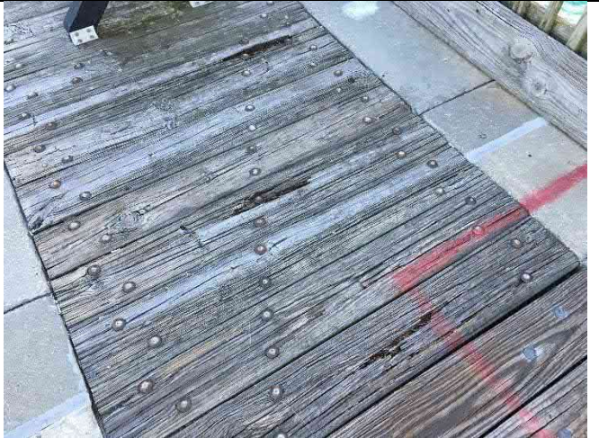
Span 24 – Deck damage
