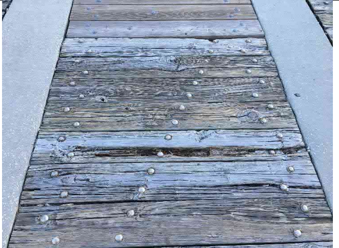
Span 26 – Damaged deck with gaps and dips > 0.5"
