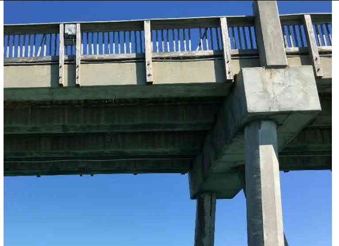
Bent 35W – Beam 34-4 South end cracking, delamination and spall 24”x4”x3”
