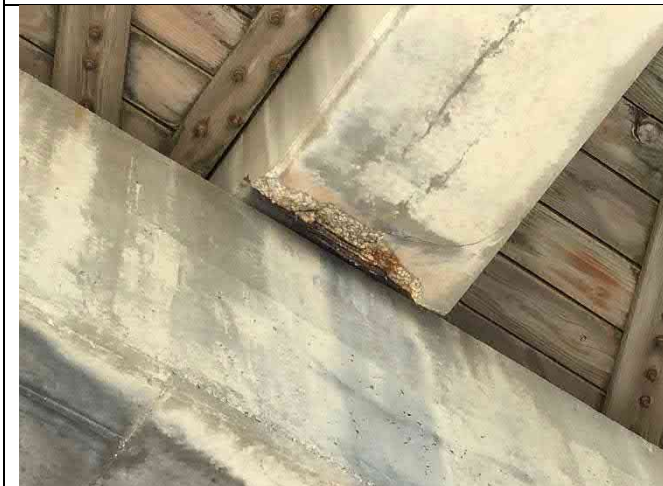
Beam 10-2 North - End cracking and spalls 24"x6"x4", longitudinal cracking
