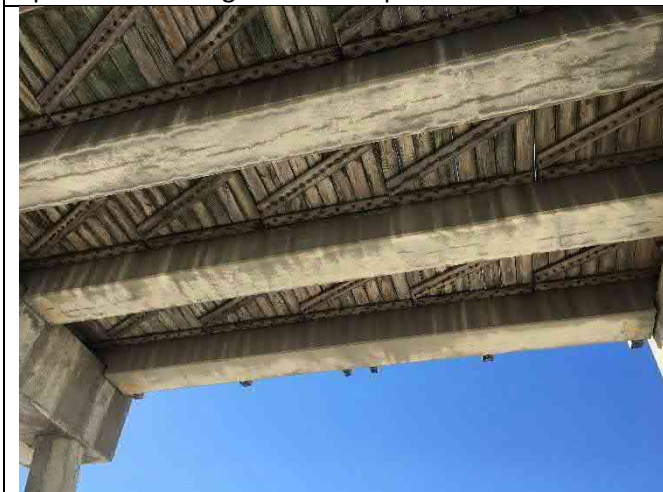
Beam 13-3 – Top flange spalls 36"x6"x1"
