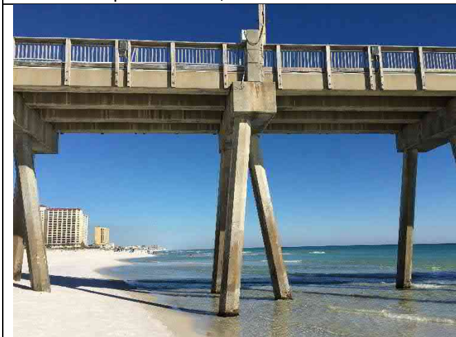
Bent 15W – Rust staining below light column, Pile 15-2 spall 4"x4"x2"
