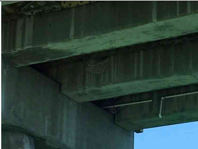
Beam 26-2 North – Spall 24”x20”x3”
