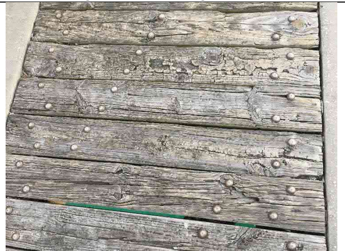
Span 40 – Deck damage with gaps and dips > 0.5"
