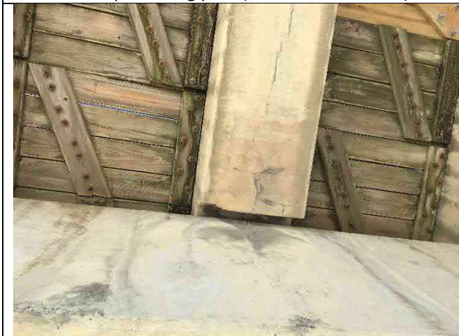
Beam 6-3 North – Small end spall, end cracking and delamination 24"x12", longitudinal cracking
