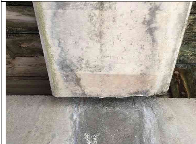
Beam 4-3 South – Bottom flange cracking, end spall and spall forming, longitudinal cracking
