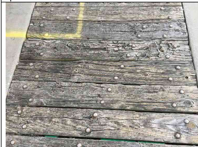
Span 40 – Deck damage with gaps and dips > 0.5"
