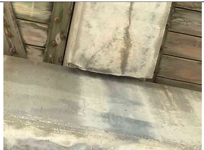
Beam 10-3 North – End cracking and spalls 24"x6"x4", longitudinal cracking
