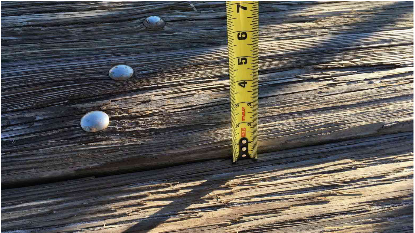
Figure 5 – Timber Deck Blowout Panel Dip > 0.5"
