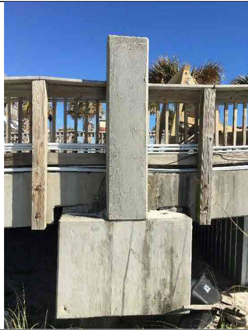
Bent 4W – Pile cap spall and closure cracking, loose railing components
