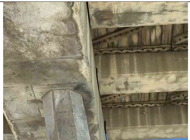
Span 14 North – Beams shifted north, end beam cracking
