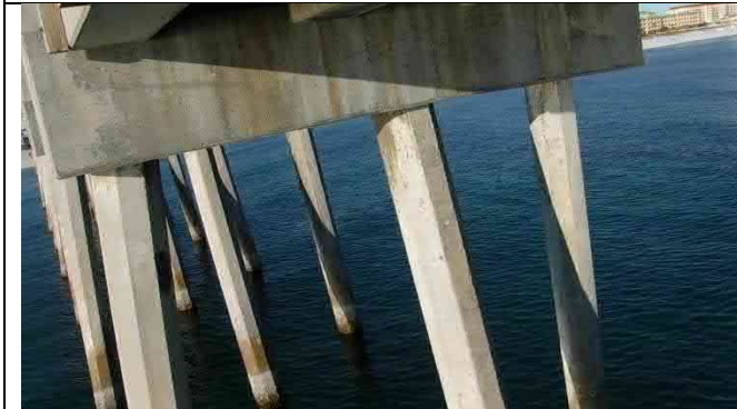
Bent 34 South Face – Beam 34-4 North end cracking and delamination 24"x6"x3"
