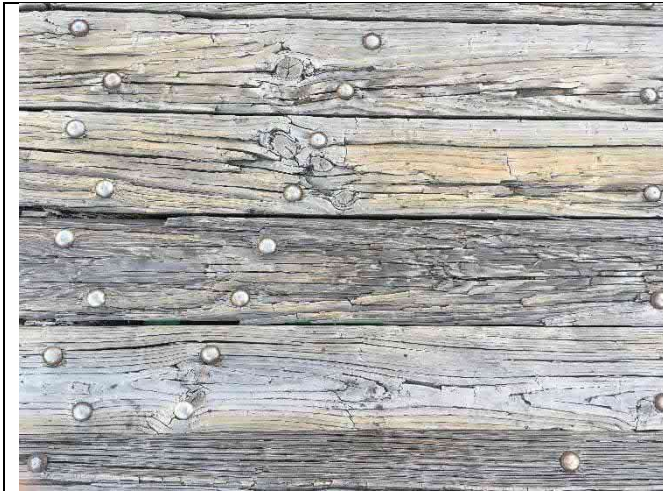
Span 34 – Deck damage with gaps and dips > 0.5"
