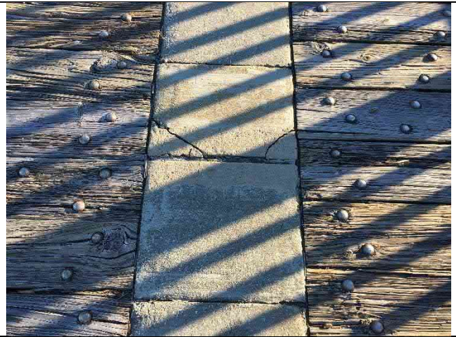
Span 8 – Closure cracking, deck deterioration
