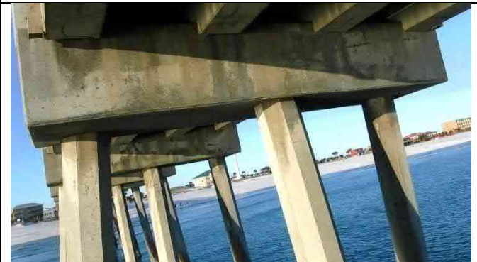
Bent 28 South Face – Beam 28-4 North end cracking, delamination and spall 24"x6"x4", Pile 28-1 top spall 10"x4"x1"
