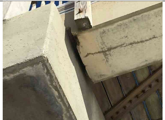
Beam 11-4 North – Spall 8"x4"x3", longitudinal cracking
