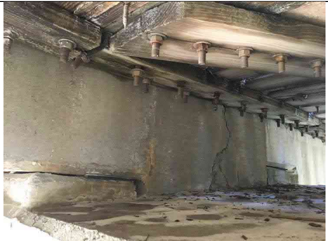
Bent 4W – Closure cracking, loose bolts
