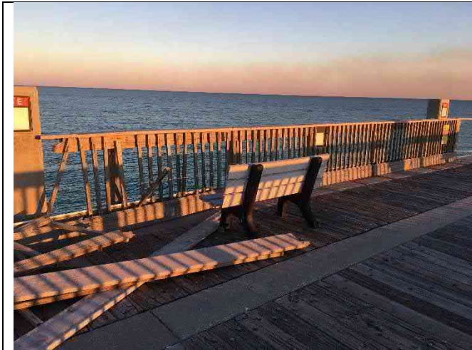
Span 33E – Railing damaged
