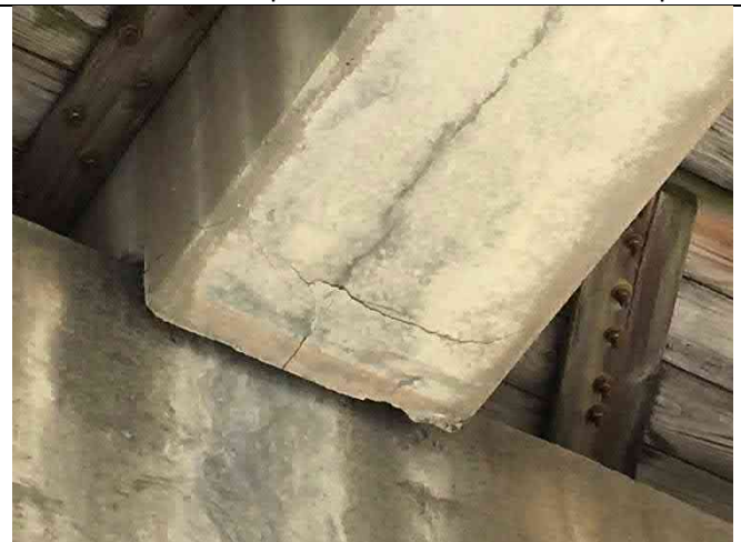
Beam 9-3 South – End cracking and delamination 24"x12"x4", longitudinal cracking
