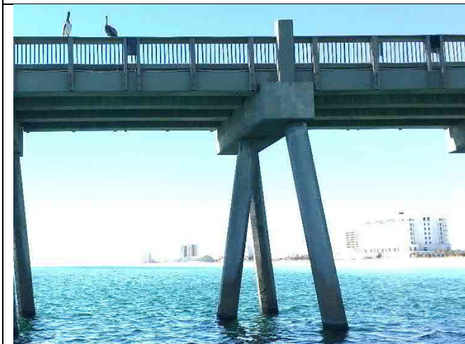
Bent 28E – Piles 28-1, 28-2, 28-3 previous spall repair damage 3x4~5"x5"x2"
