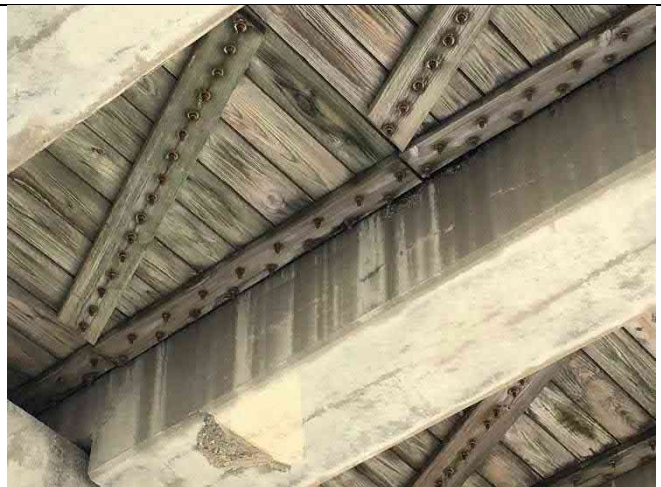
Beam 12-3 South – End cracking and spall 36"x24"x2", top flange spalls 36"x3"x2", longitudinal cracking
