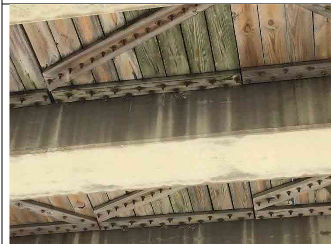
Beam 11-3 – Top flange spalls 12”x6”x2”
