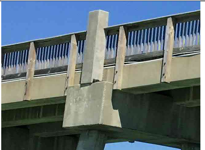
Bent 20W – Light column spall 12"x3"x3"
