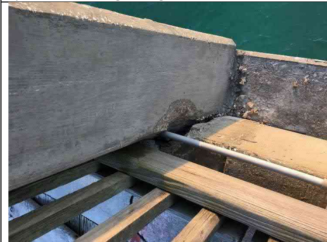
Bent 23W – Light column spall 14"x6"x4"
