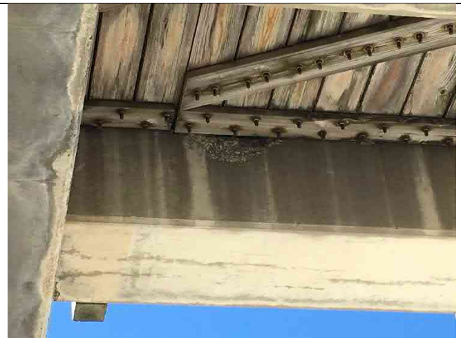
Beam 9-4 South – Spall 20"x12"x3" from deck impact
