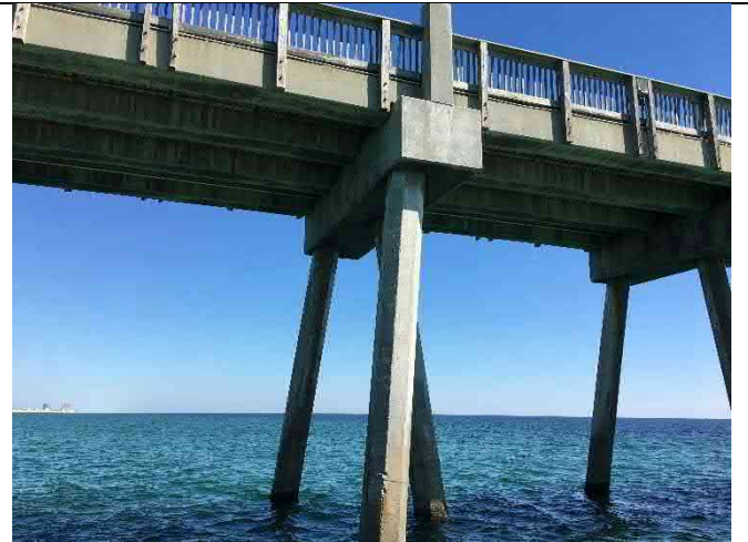
Bent 41W – Pile spall repair damage 3x4~4"x4"x2"
