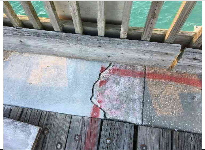
Bent 23W – Closure cracking
