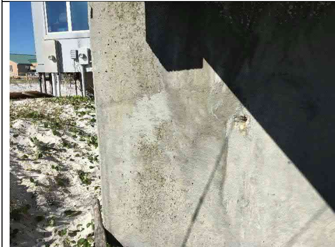
Bent 4W South – Cap spall 2"x2"x1"
