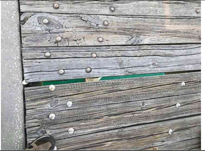
Span 36 – Deck damage with gaps and dips > 0.5"
