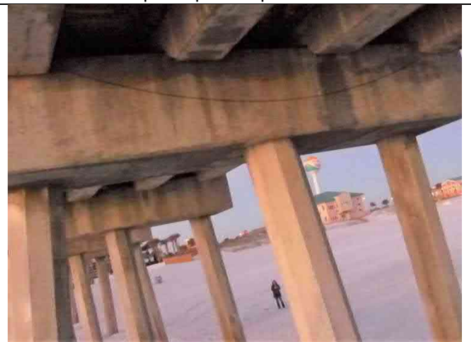
Bent 15 South Face – Beam 15-3 North end cracking and delamination
