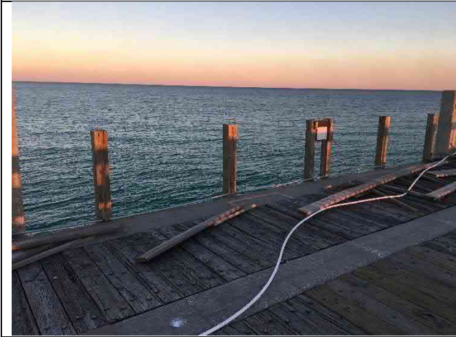
Span 36E – Railing destroyed, utility damage
