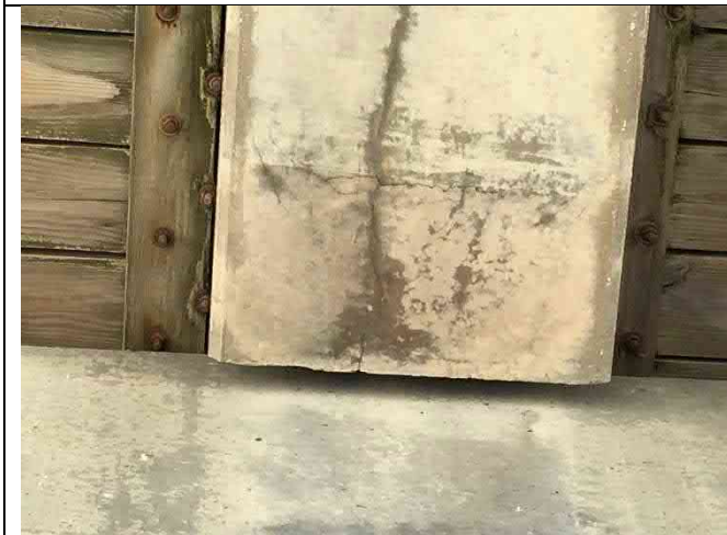
Beam 8-2 North – End cracking and delamination
