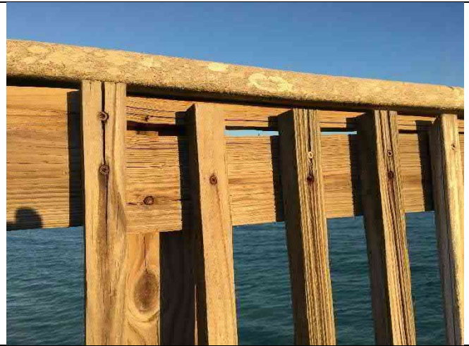
Span 21E – Typical railing split wood for section still connected
