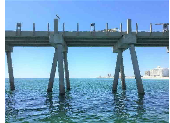
Bent 31E – Pile spall repairs damaged 3x4~4"x4"x1"
