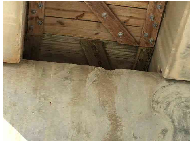
Bent 7 South Face – Spall 8"x4"x2"
