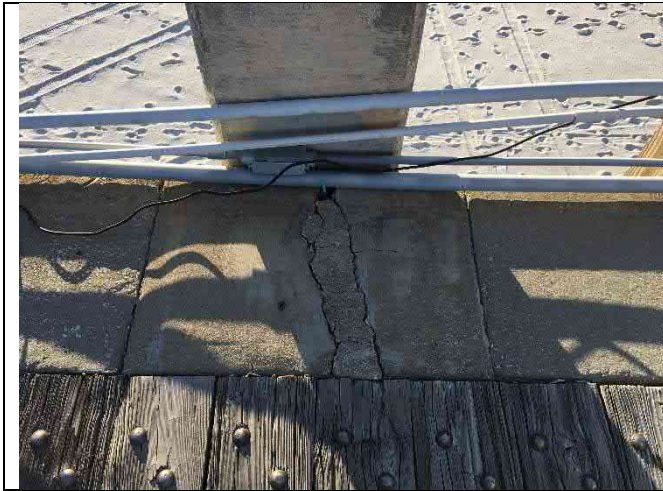
Bent 10W – Closure cracking
