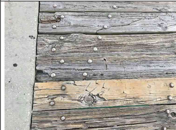
Span 38 – Deck damage with gaps and dips > 0.5"
