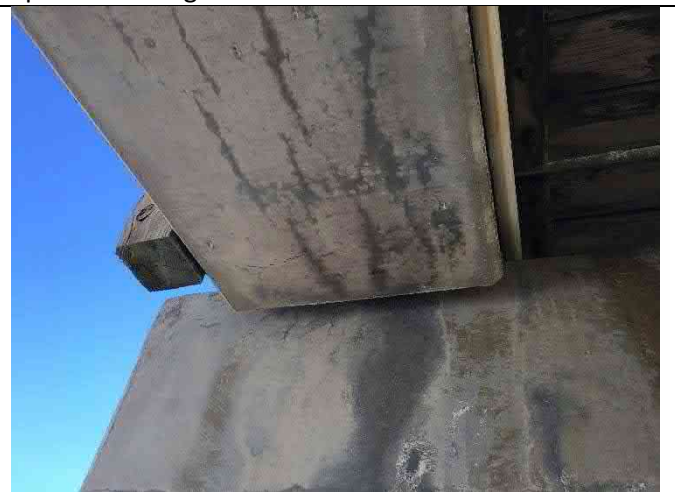
Beam 4-1 South – Bottom flange cracking, end delamination and spall forming, longitudinal cracking
