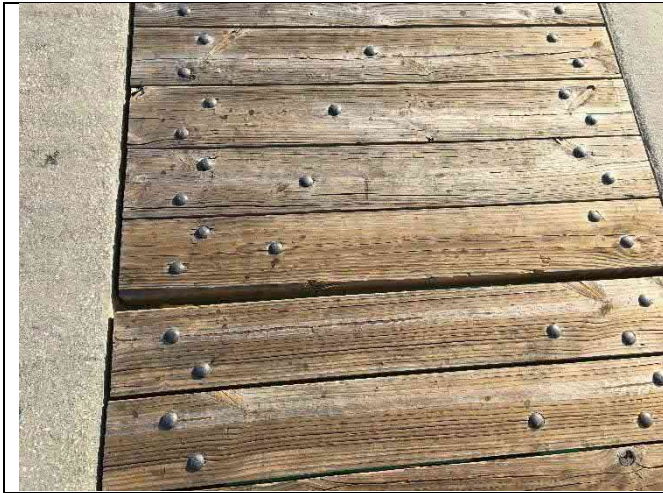
Span 47 – Deck damage with gaps and dips > 0.5"
