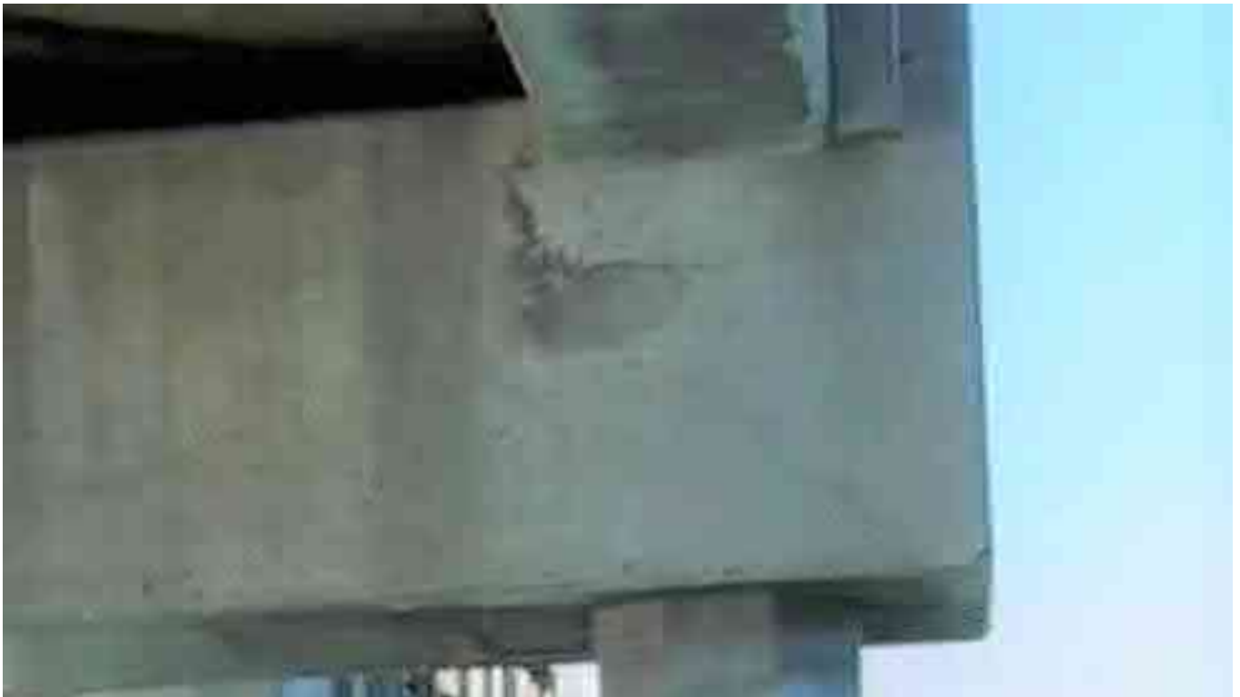
Figure 17 – Pile Cap Spall from Impact
