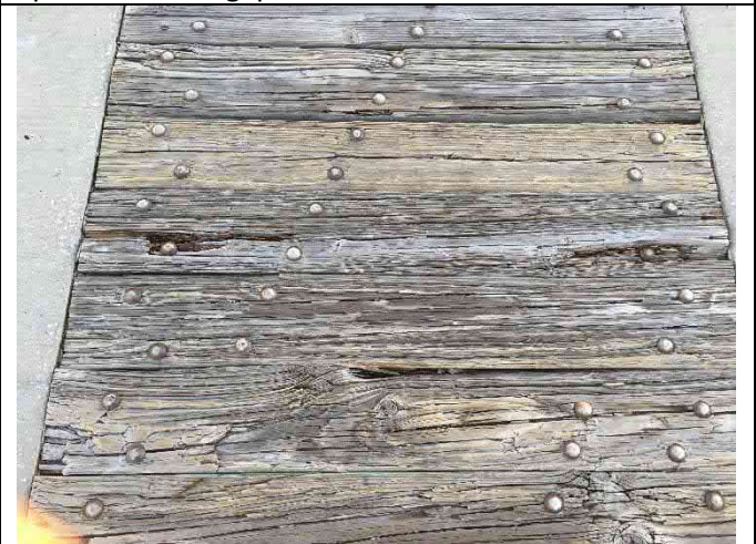
Span 34 – Deck damage with gaps and dips > 0.5"
