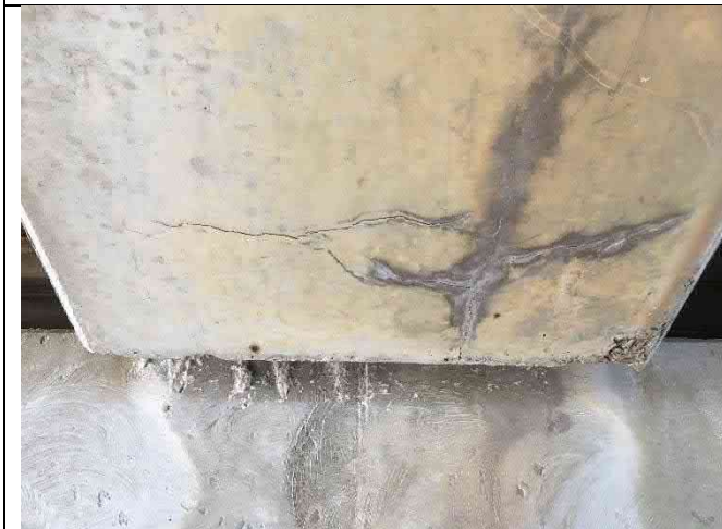
Beam 4-2 North – Bottom flange cracking, spall forming, longitudinal cracking
