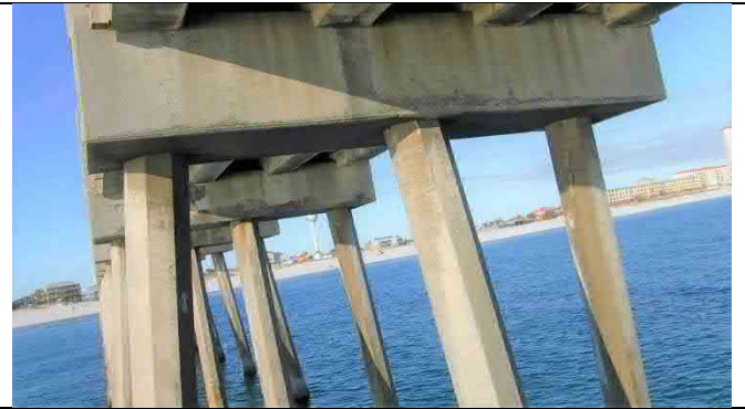
Bent 40 South Face – Pile 40-1 top spalls 15"x3"x1", 8"x8"x2"
