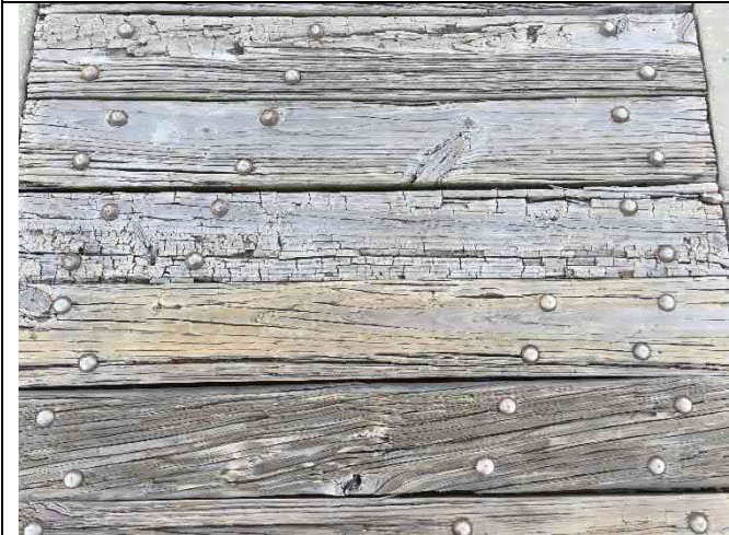
Span 35 – Deck damage with gaps and dips > 0.5"
