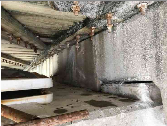
Bent 4 Center – Closure cracking, loose bolts
