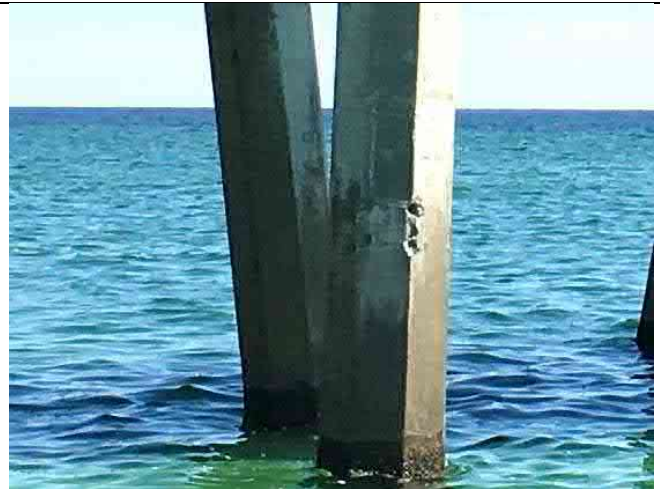
Pile 24-3 – Pile repair partially damaged 4~5"x5"x1"
