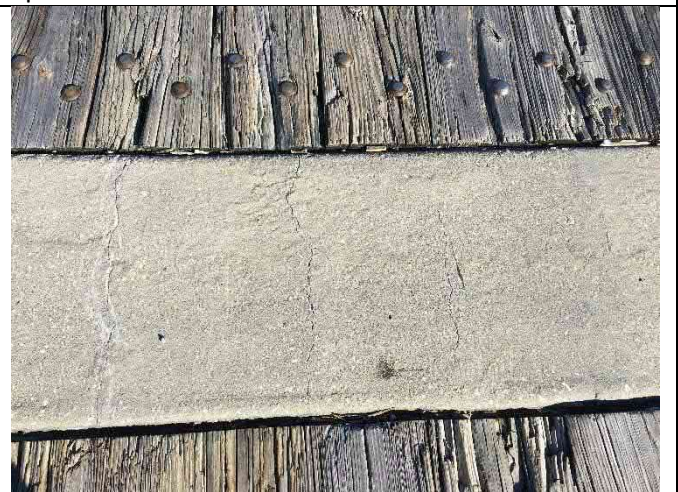
Beam 20-2 and 20-3 – Top flange cracking 12" +/- on center full length
