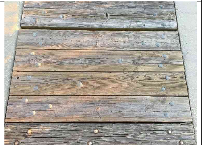
Span 34 – Deck gaps > 0.5"
