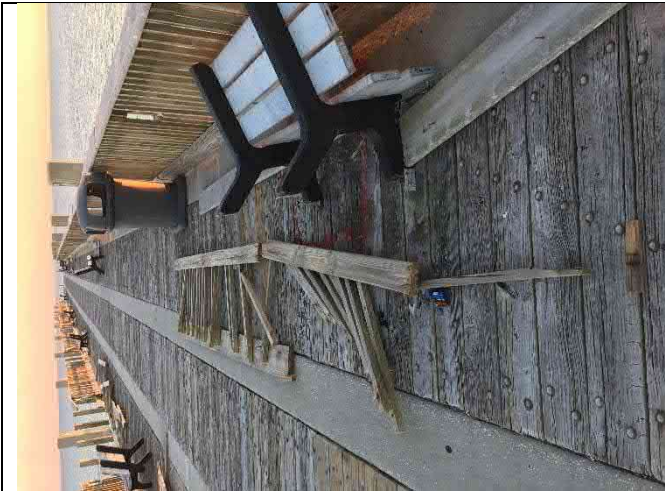
Span 36W – Bench to deck connection damage
