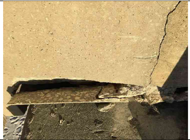
Beam 9-4 South – Spall 16"x4"x4", closure spall 14"x4"x4"
