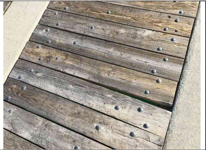
Span 47 – Deck damage with gaps and dips > 0.5"
