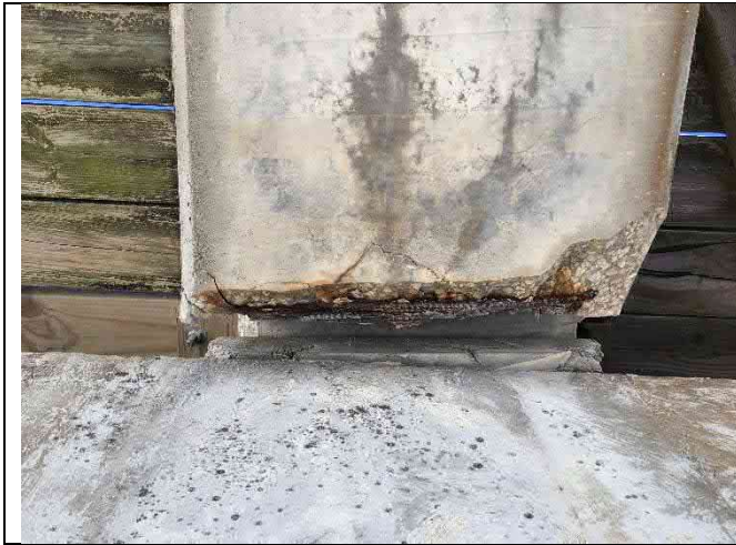
Beam 5-2 North – Cracking and spall 24"x6"x4" bottom flange, longitudinal cracking, spalls on dapped end 16"x8"x1" each side
