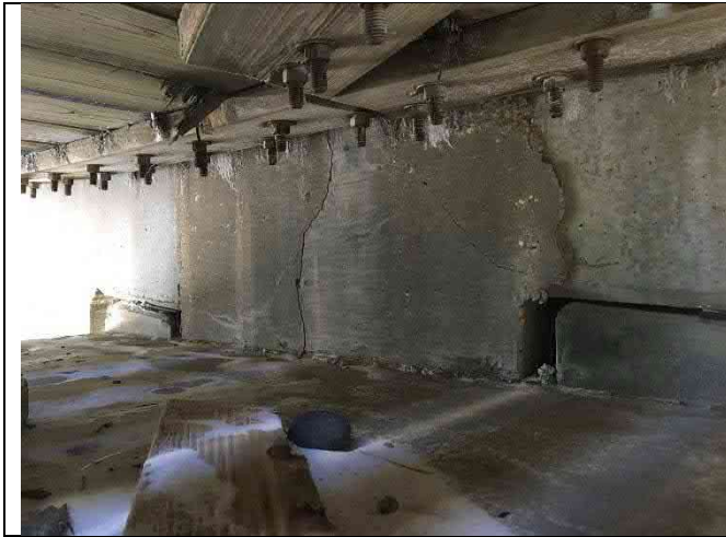
Bent 4 Center – Closure cracking
