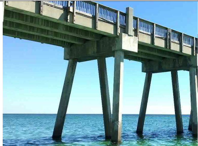
Bent 24W – Pile 24-3 repair partial damage 4~5"x5"x1"
