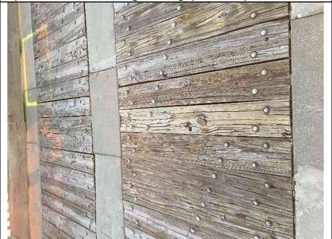
Span 38 – Deck damage with gaps and dips > 0.5"
