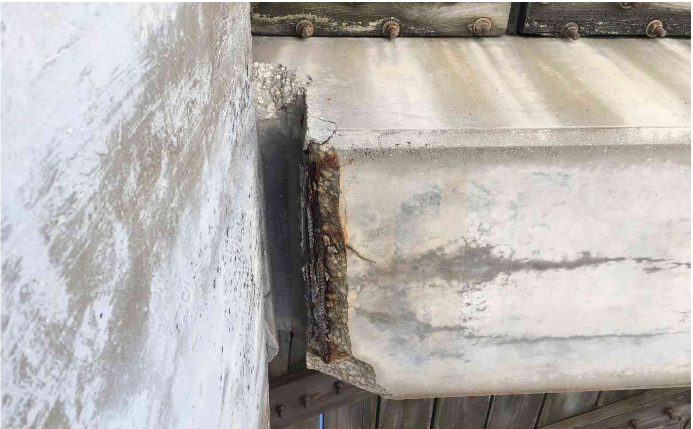
Figure 14 – Typical Beam End Cracking and Spall
