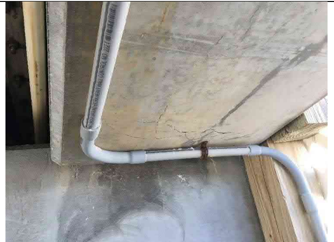
Beam 4-1 North – Bottom flange cracking and spall forming, longitudinal bottom flange cracking
