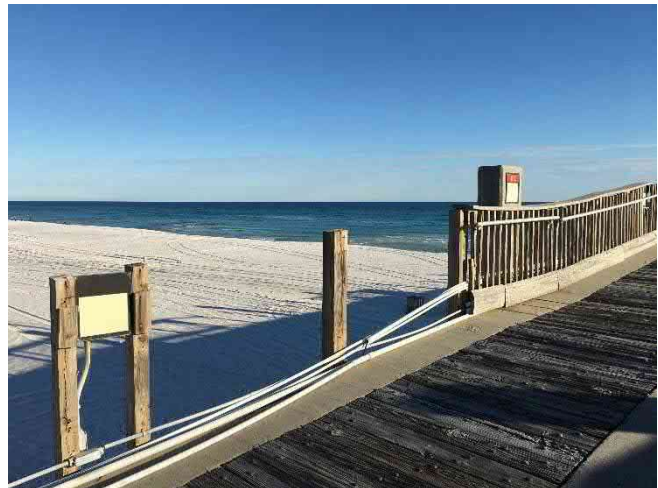
Span 5E – Missing railing (guardrail and handrail)
