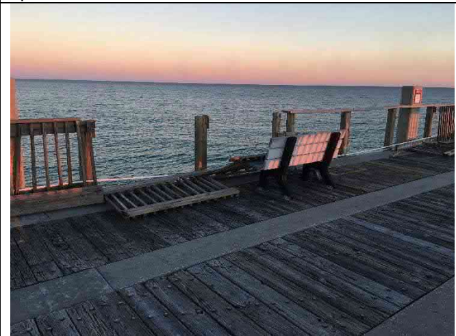
Span 41E – Railing damage
