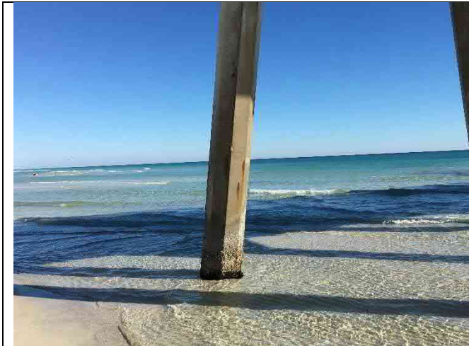
Pile 15-1 – Spall 5"x3"x2", rust stains
