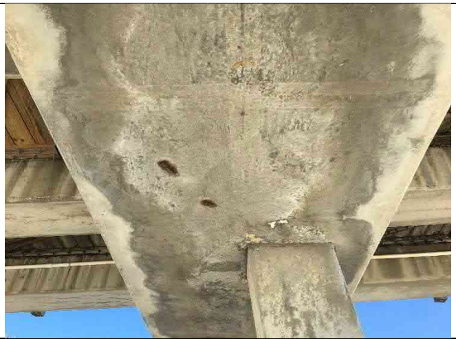
Bent 6 – Pile cap minor spalls and rust from exposed reinforcement or chairs
