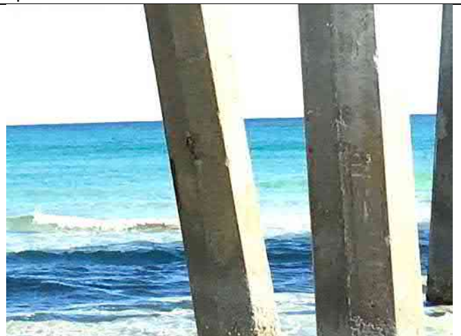
Pile 16-2 – Spall 12"x5"x2"
