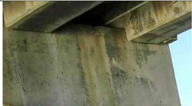
Bent 34 South Face – Pile cap top spall 8"x6"x1"
