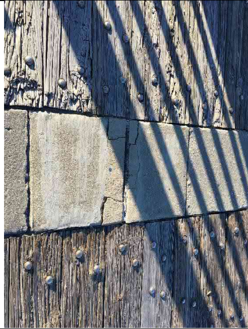
Bent 6 – Closure cracking
