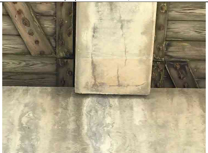
Beam 14-2 South – End beam cracking and delamination
