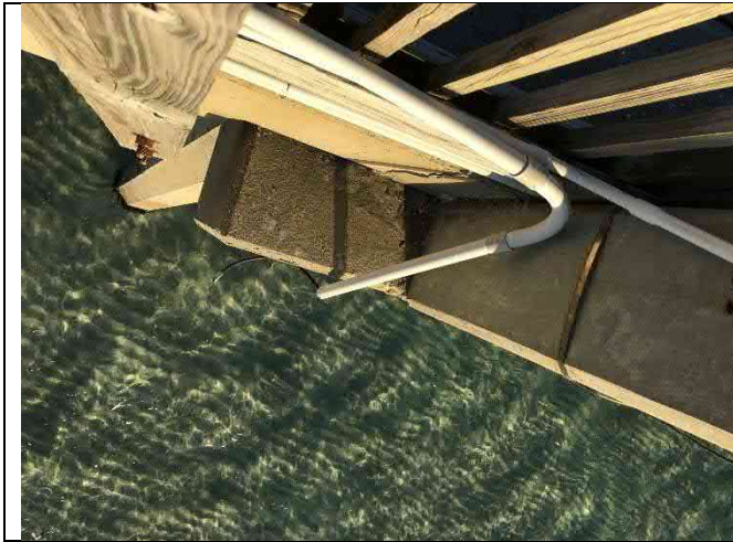
Bent 15W – Closure cracking, utility damage
