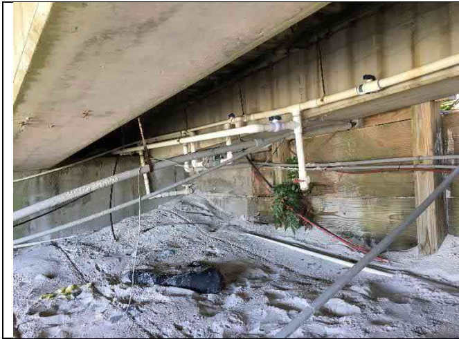
Bent 3E – Water and electrical conduit damage
