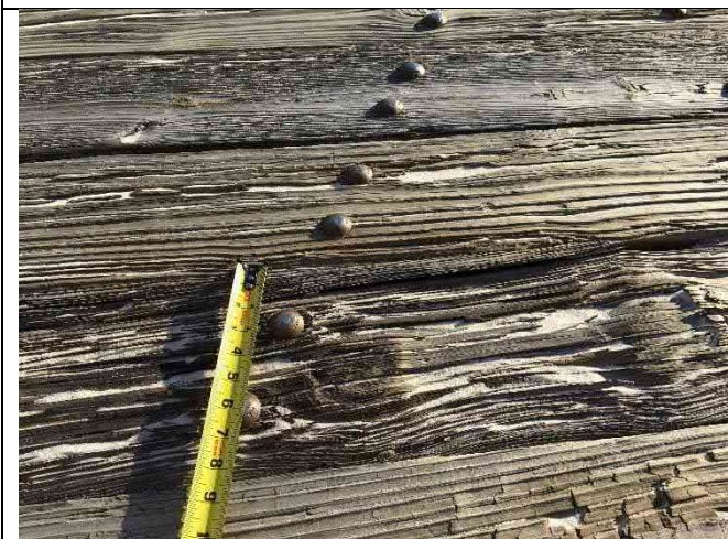
Span 4 – Rough deck surface with changes in elevation between 0.25" and 0.5" without bevel and greater than 0.5" exceeding ADA 4.5.2 limits.
