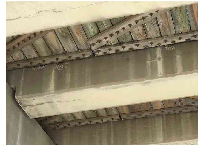
Beam 11-3 North – Top flange spalls 24"x8"x2" total, beam end cracking
