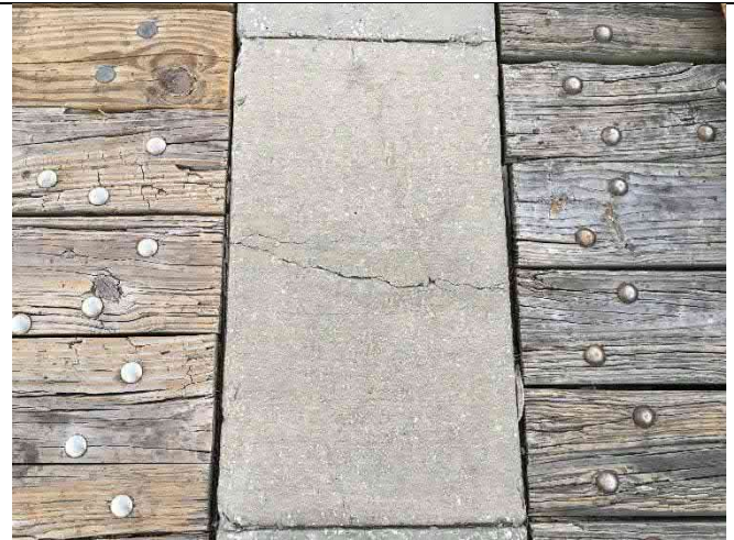
Bent 43 – Closure cracking
