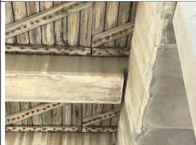
Beam 8-3 South – End spall 4"x4"x2", longitudinal cracking
