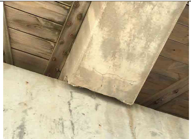
Beam 7-2 North – End cracking and delamination, spall 24"x2"x3"
