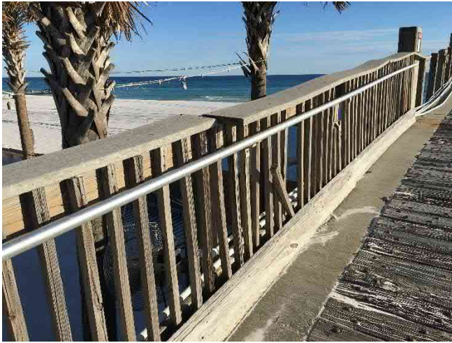
Span 4E – Railing damage and loose components
