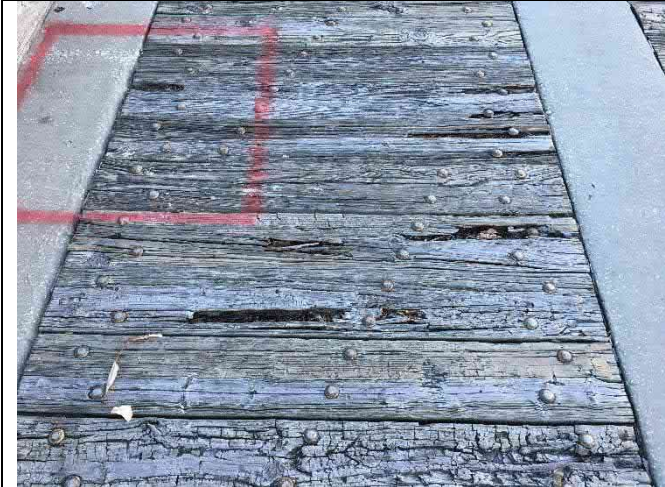
Span 26 – Damaged deck with gaps and dips > 0.5"
