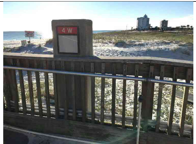
Bent 4W – Loose railing components
