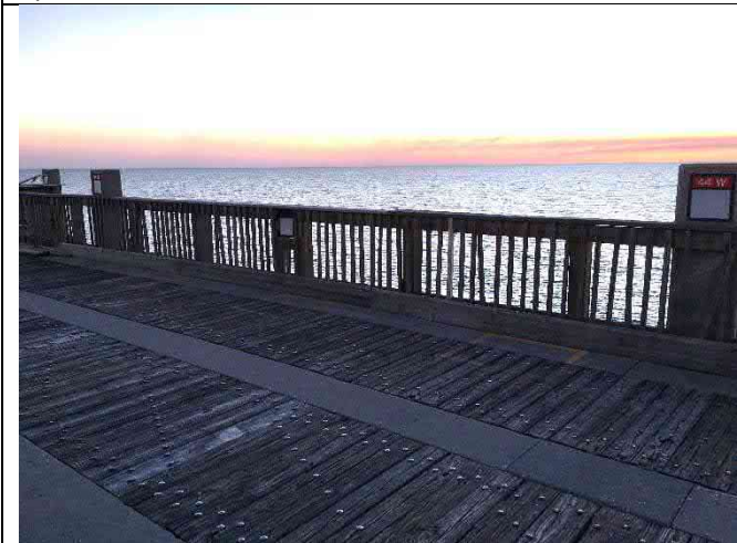
Span 44W – Railing loose with split wood members
