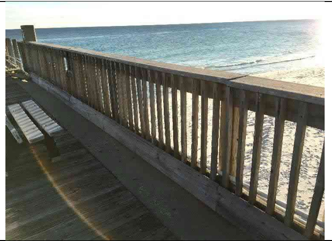
Span 12W – Railing loose with split wood
