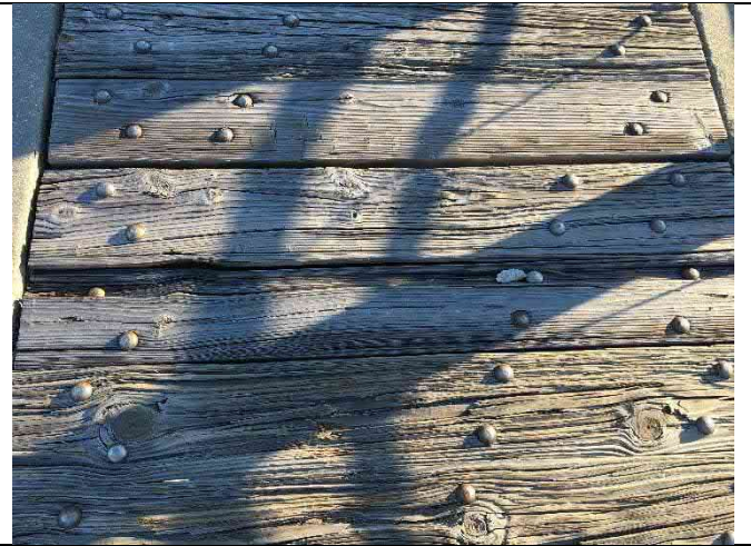
Span 9 – Deck damage with gaps and openings exceeding 0.5"
