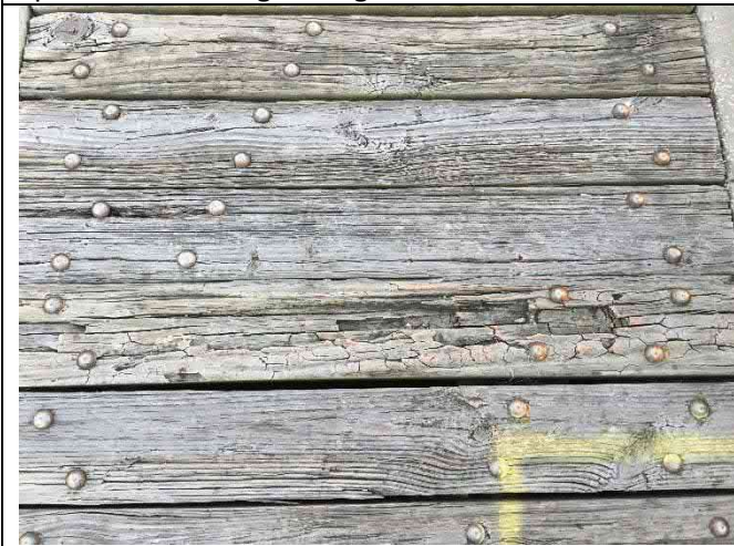
Span 39 – Deck damage with gaps and dips > 0.5"
