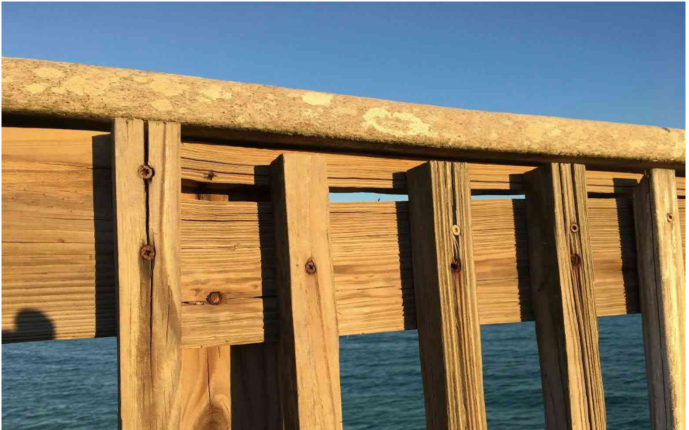
Figure 9 – Pedestrian Railing Loose and Split Timber Members
