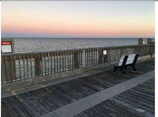
Span 44E – Railing loose with split wood members
