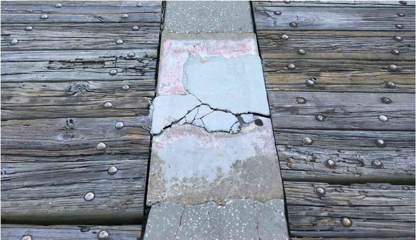
Figure 13 – Typical Closure Pour Cracks and Spalls
