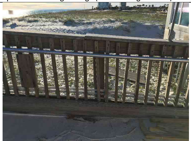
Span 3W – Loose and damaged railing components
