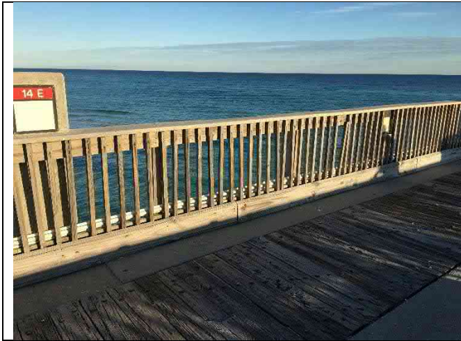
Span 14E – Railing loose with split wood members
