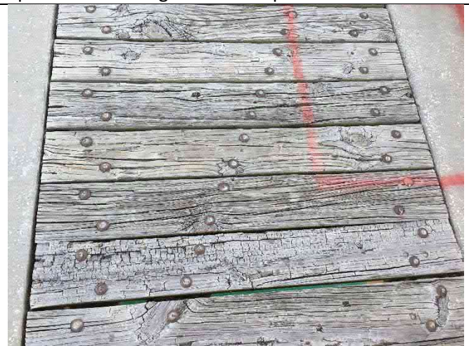
Span 33 – Deck damage with gaps and dips > 0.5"
