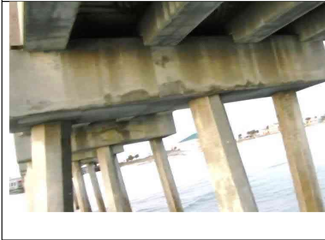
Bent 19 South Face – Beam end cracking (common)
