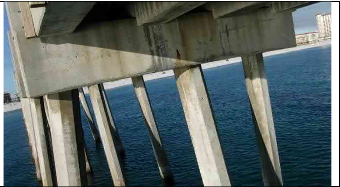
Bent 37 South Face – Pile cap spall with rust staining 3"x3"x2"
