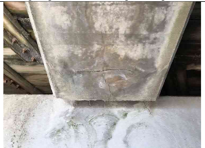
Beam 4-3 North – Bottom flange cracking, spall forming, longitudinal cracking
