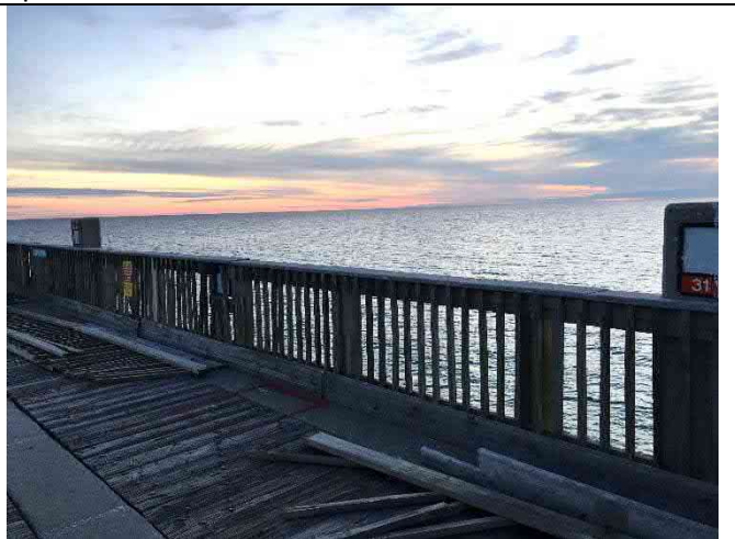
Span 31W – Railing loose with split wood members
