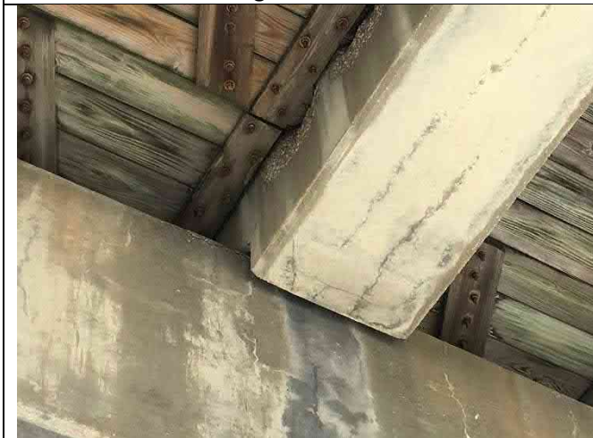
Beam 11-3 South – End cracking and delamination, pile cap cracks
