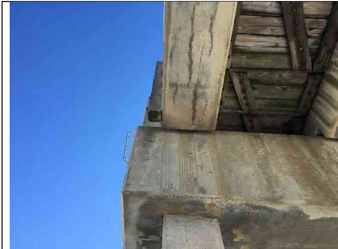
Beam 6-1 South – End cracking and delamination
