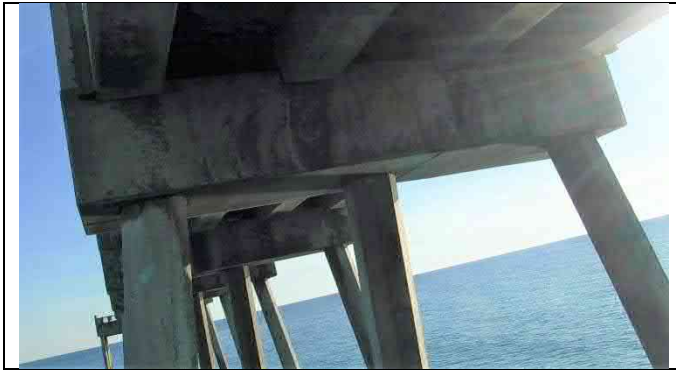
Bent 37 North Face – Pile 37-1 top spall 4"x4"x1"
