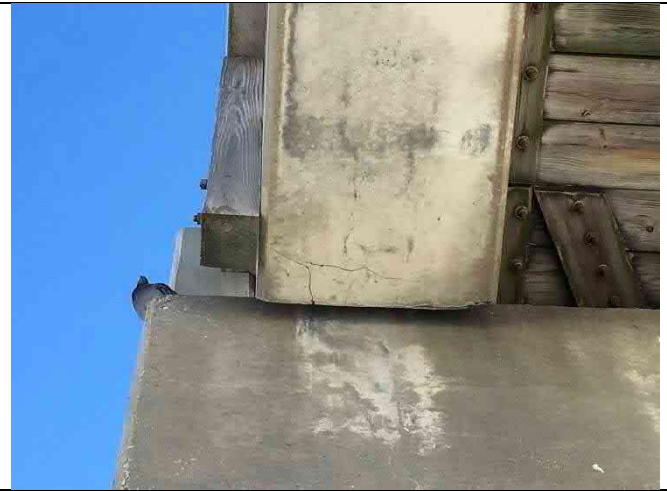
Beam 11-1 South – End cracking and delamination
