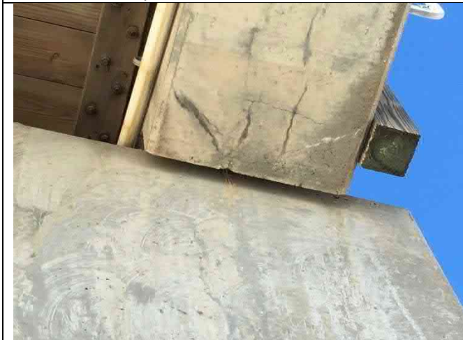
Beam 7-1 North – End cracking and delamination, longitudinal cracking
