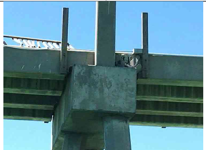
Beam 22-1 South – Spall 16"x16"x6", closure spall 16"x12"x6"
