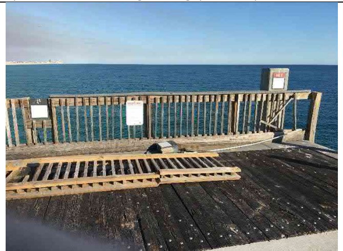
Span 47E - Deck and railing damage
