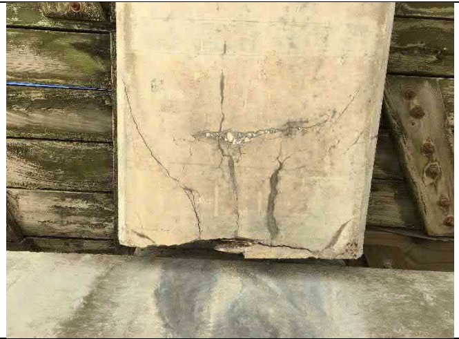
Beam 5-3 North – End cracking, delamination and spall 24"x24"x1", longitudinal cracking
