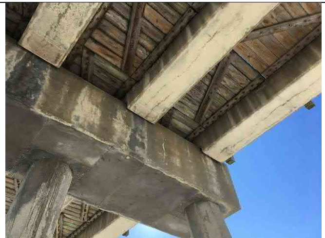
Bent 12 North Face – Pile cap cracks (30' +/-), spall 5"x5"x1"
