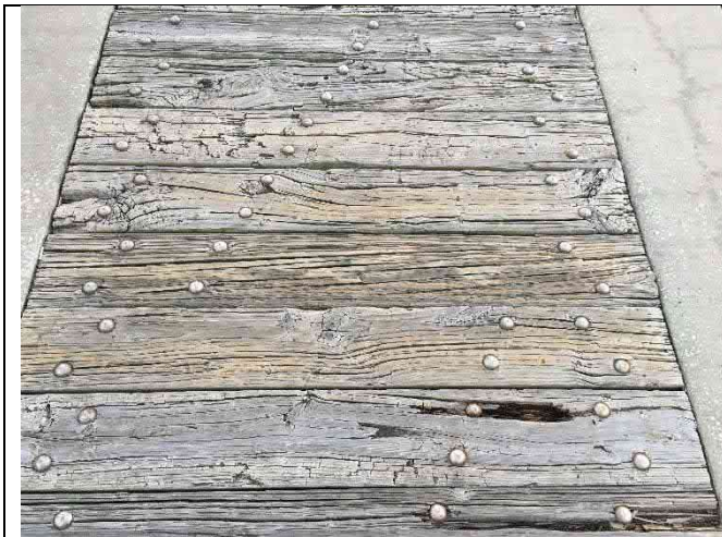
Span 39 – Deck damage with gaps and dips > 0.5"
