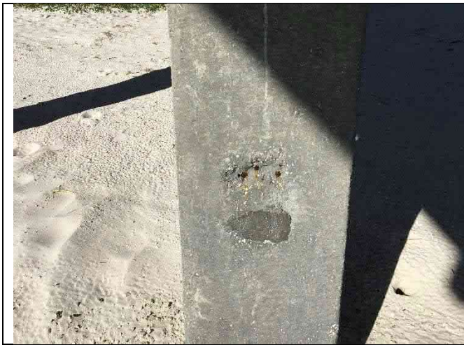
Pile 6-2 – Spall 7"x4"x1"
