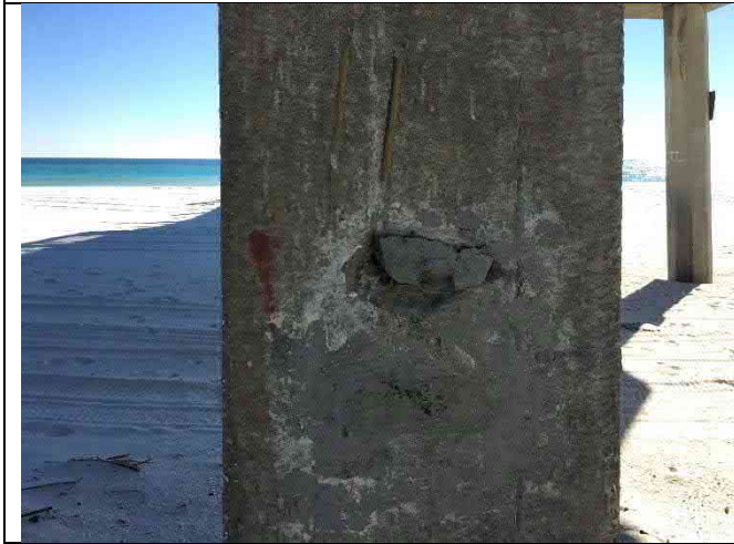
Pile 7-1 – Spall 8"x5"x2"
