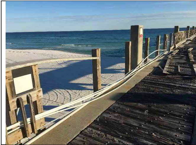
Span 7E – Damaged and missing railing
