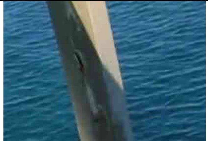
Pile 27-1 – Spall 12"x5"x2"
