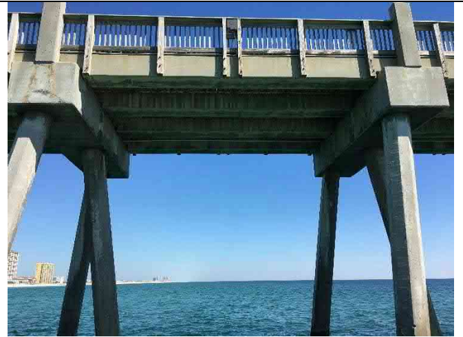
Bent 39W, 40W – Pile 40-1 top spalls, Pile 40-3 spall repairs damaged 4~4"x4"x2"
