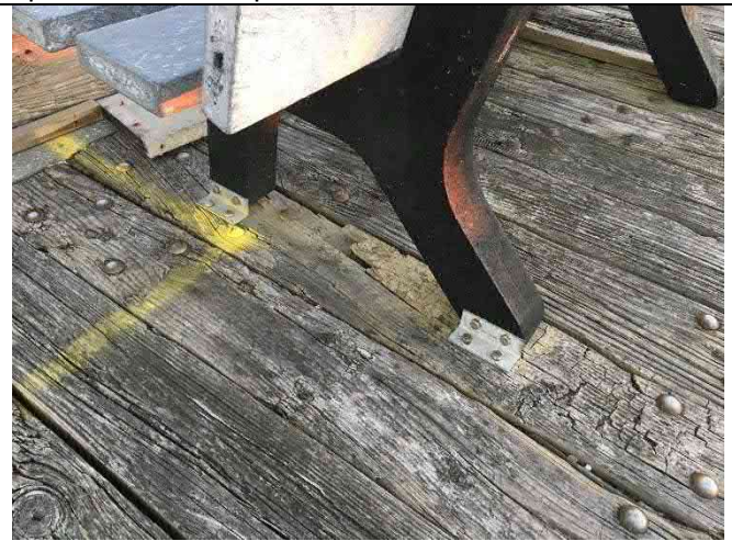
Span 39 – Broken deck below bench
