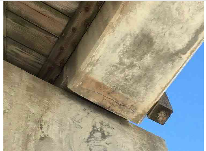
Beam 6-4 South – End cracking and delamination
