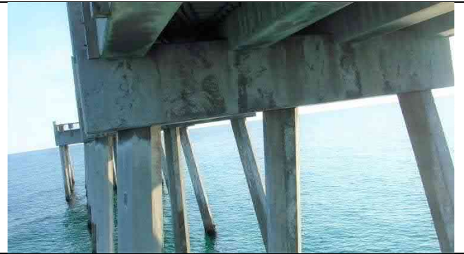
Bent 41 North Face – Pile 41-1 top spall 8"x3"x1", Beam 40-1 South end cracking and delamination 24"x6"x3"
