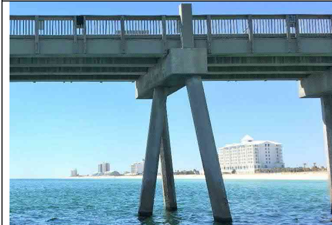
Bent 27E – Spall repairs damaged all piles 3x4~4"x4"x1"
