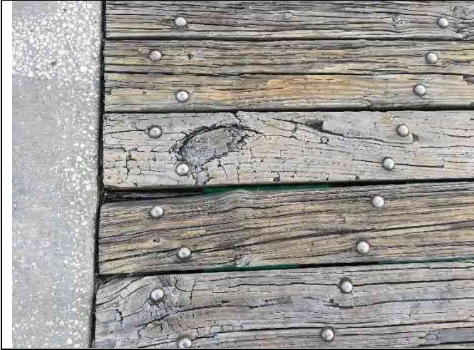
Span 36 – Deck damage with gaps and dips > 0.5"
