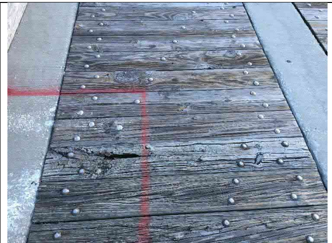
Span 28 – Timber deck deterioration
