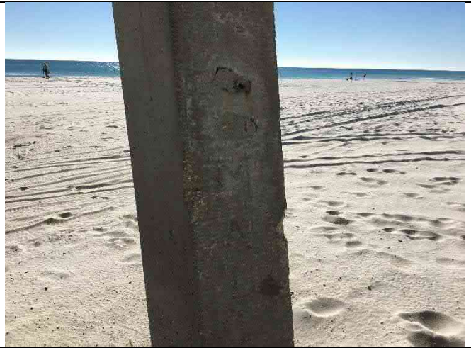
Pile 7-3 – Multiple spalls, 22"x3"x2"
