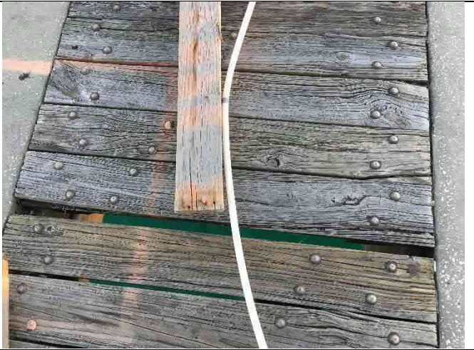
Span 36 – Deck damage with gaps and dips > 0.5"
