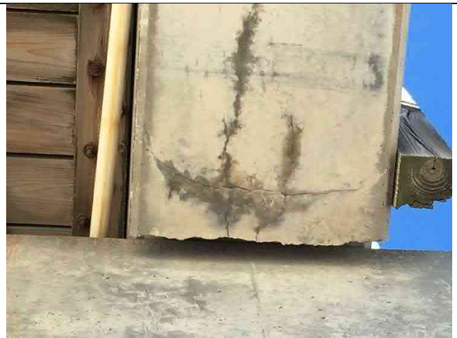
Beam 8-1 North – End cracking and delamination and spall 24"x12", longitudinal cracking
