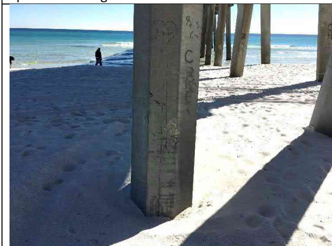
Pile 12-1 – Spall 12”x6”x2”
