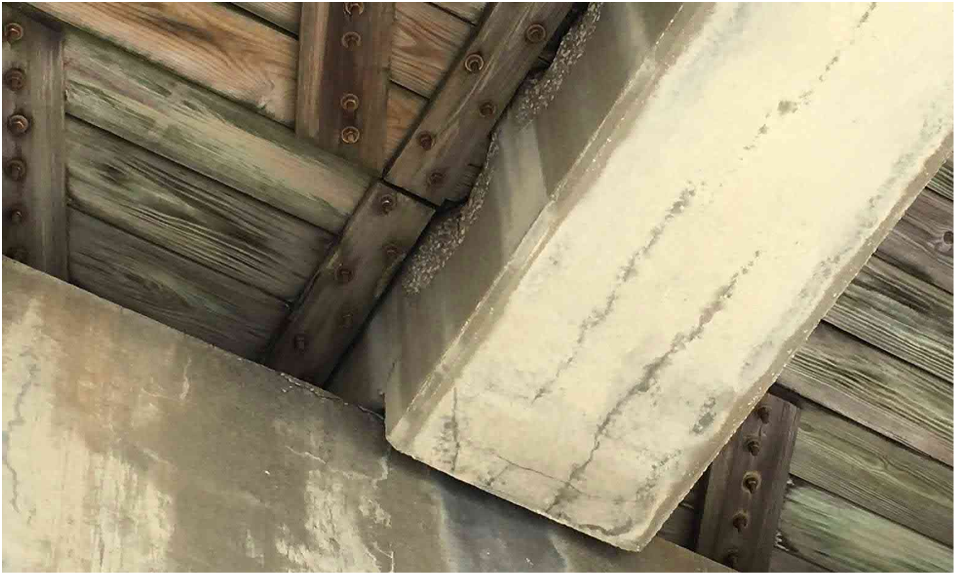
Figure 15 – Typical Beam Top Flange Spall
