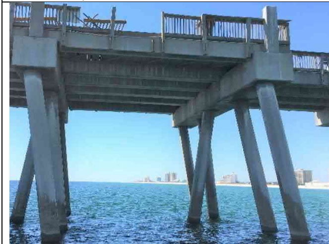
Bent 46E South Face – Pile spall repairs damaged 5x4~4"x4"x1"
