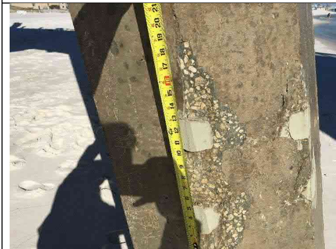
Pile 14-2 – Spalls 20"x10"x2", 16"x5"x2"
