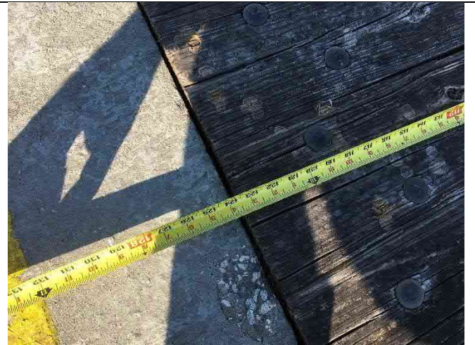
Beam 74-2 – Top flange spall 4"x2"x1"
