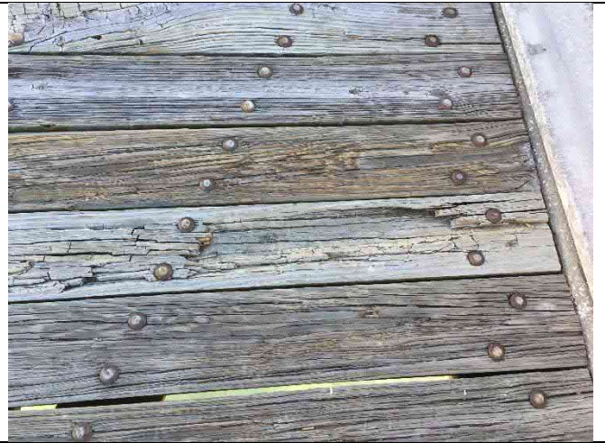
Span 16 – Deck damage with dips and gaps > 0.5"
