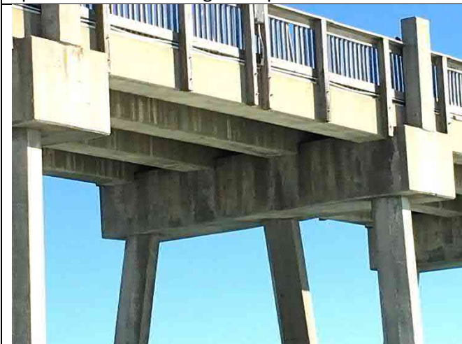
Span 18 – Bottom flange end cracking (common)
