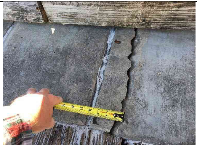
Bent 5W – Closure spall and cracking
