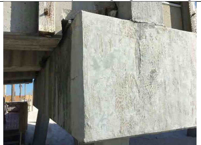
Bent 5W – Cracking (20' +/-)
