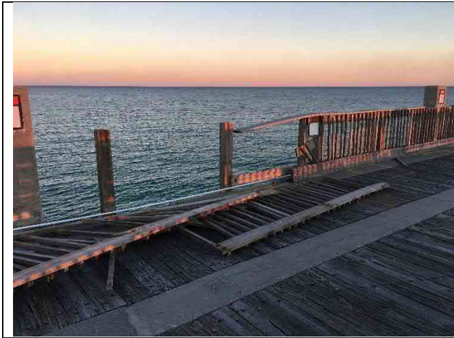
Span 38E – Railing damage
