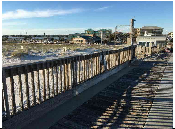
Span 7W – Railing damage – Standing railing loose with multiple wood splitting (common condition)
