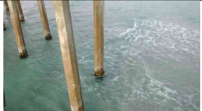
Piles 19-1 and 19-2 – Spalls 2~5"x5"x2" each
