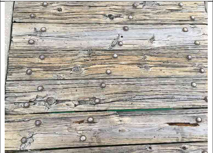
Span 38 – Deck damage with gaps and dips > 0.5"
