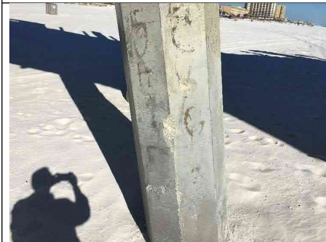
Pile 10-2 – Spalls 5"x5"x2", 12"x5"x2"
