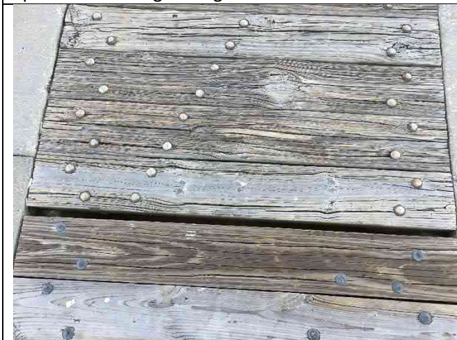
Span 33 – Deck damage with gaps and dips > 0.5"
