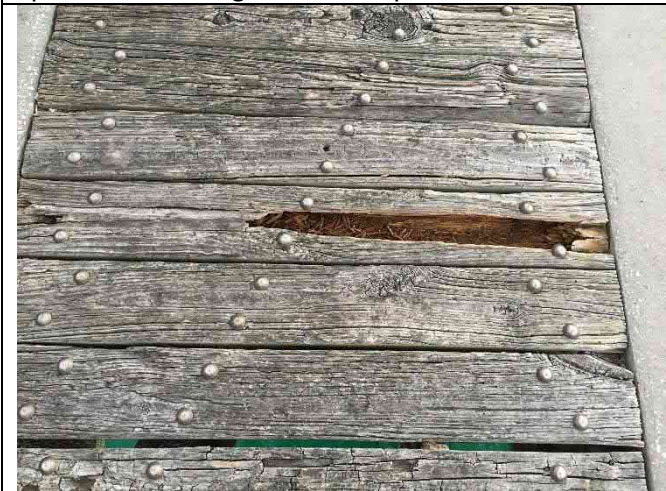
Span 44 – Deck damage with gaps and dips > 0.5"
