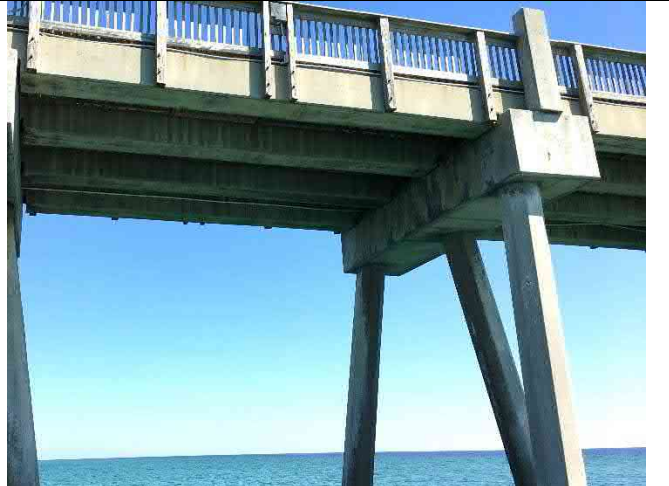
Bent 31W North Face – Pile cap spalls 2~4"x4"x2", minor rust stain under light column
