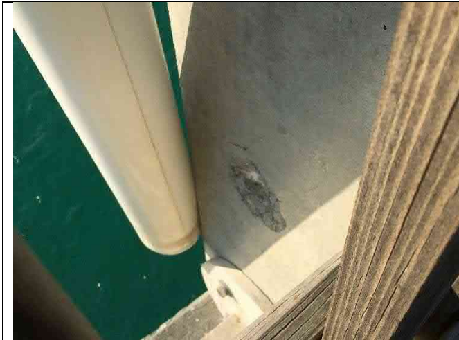
Bent 46W – Light pole column spall 5"x5"x1"
