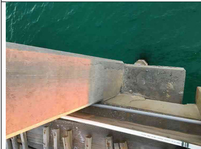
Bent 42E – Beam 42-1 closure cracking (16" +/-), light column cracking (5' +/-)
