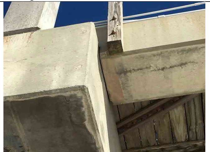
Beam 9-4 North – End spalls 8"x2"x2" combined, beam has moved north with gap closed
