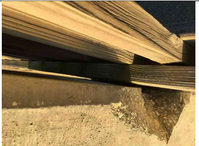
Bent 17W – Light column spall 12"x8"x4"
