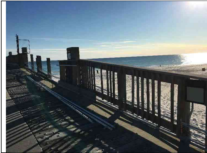
Span 5W – Missing and damaged railing
