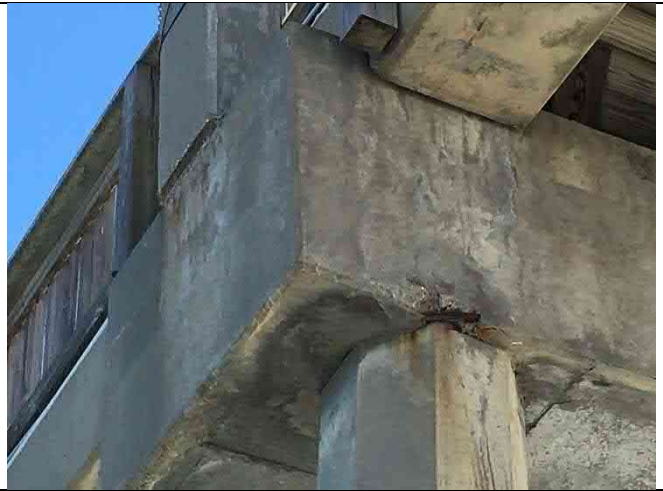
Bent 15 – Pile cap spall 14"x3"x2", hairline crack
