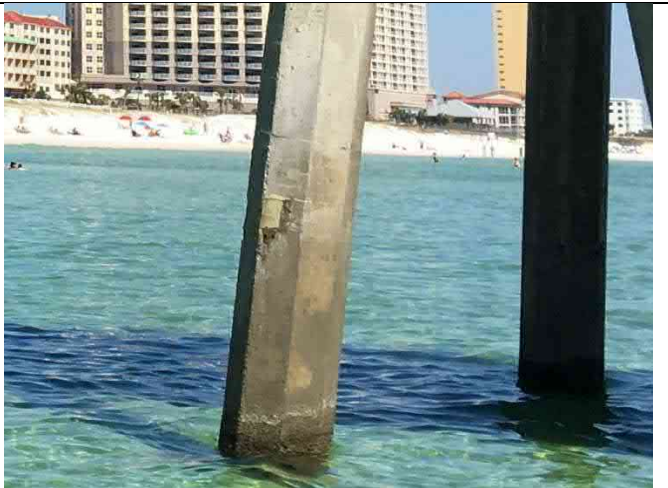
Pile 22-3 – Repaired spall
