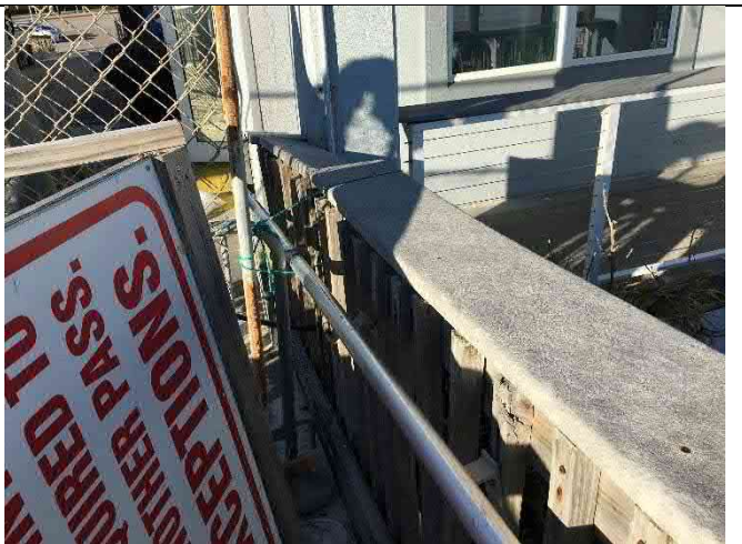
Span 3E – Railing damage (25’ of railing from B4)
