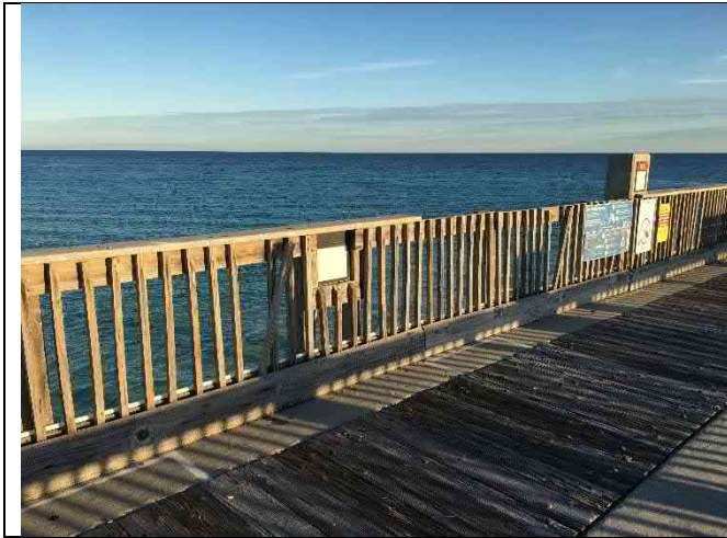
Span 16E – Railing damage
