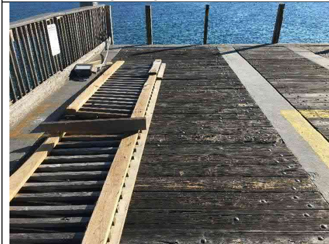
Span 47E – Deck and railing damage
