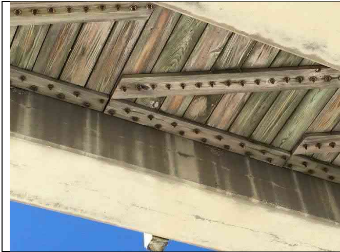
Beam 11-4 – Top flange spalls 36"x4"x1", longitudinal and horizontal cracking
