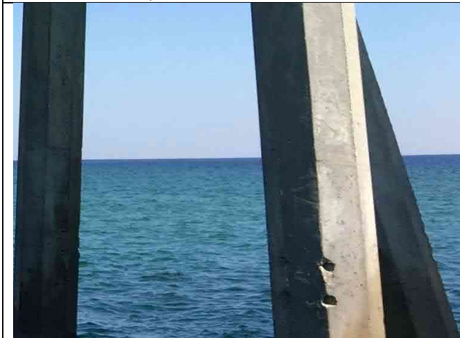
Pile 34-3 – 4~5"x5"x2" spalls (previous repair damaged)
