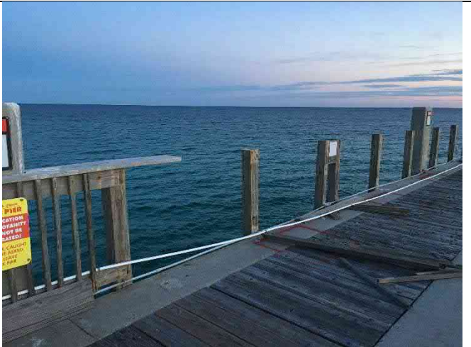
Span 34E – Railing damage
