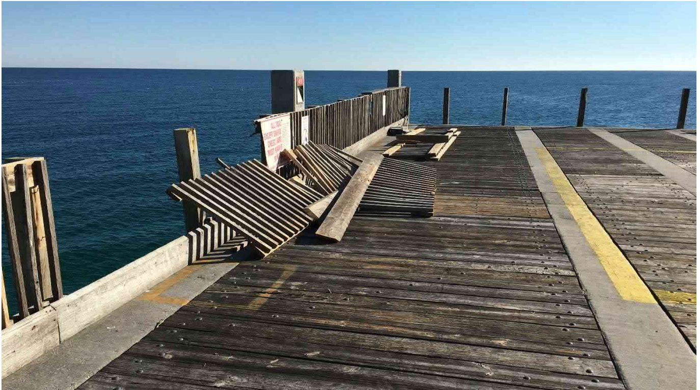
Figure 8 – Pedestrian Railing Destroyed End Spans
