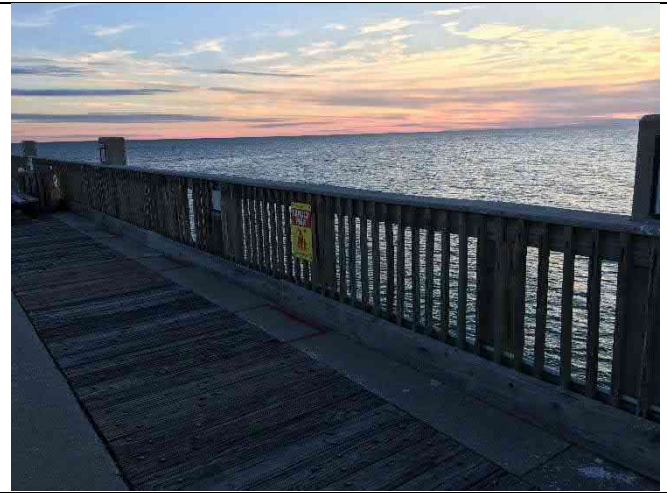
Span 27W – Railing loose with split wood members
