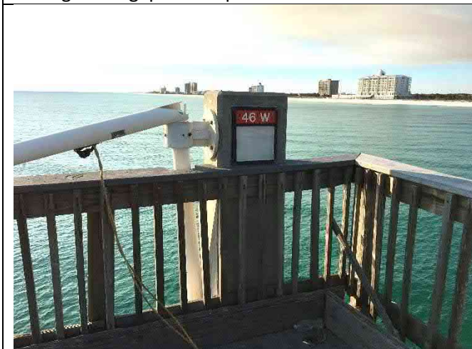
Bent 46W – Broken flagpole, railing damage
