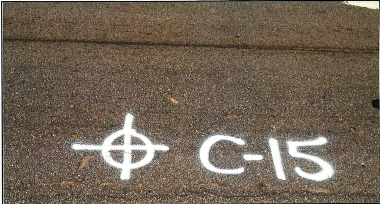
Photo 29: Alligator cracking, longitudinal cracking, rutting in wheel paths, and weathering and raveling.
