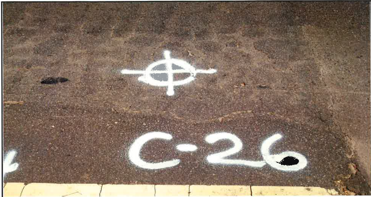
Photo 51: Alligator cracking, rutting, weathering, pumping of soil fines.
