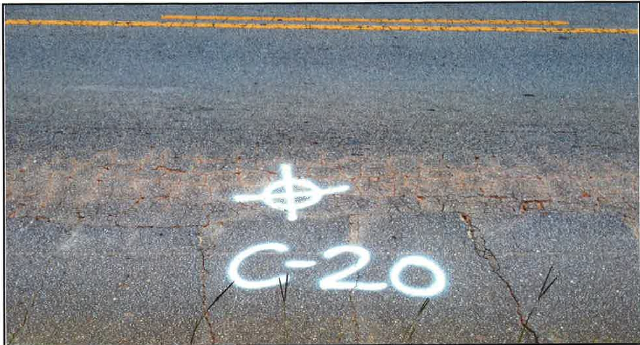
Photo 39: Alligator cracking, rutting in wheel paths, block cracking and pumping of soil fines.
