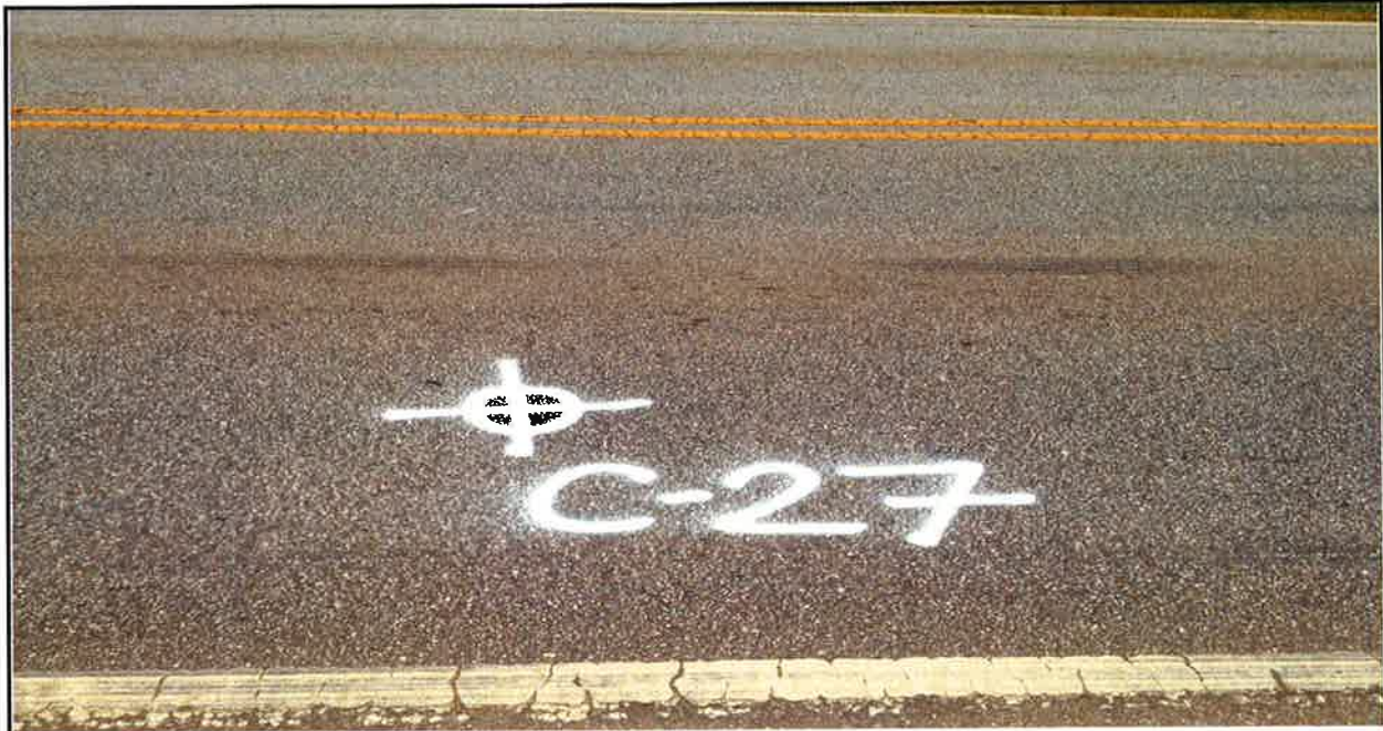
Photo 53: Minor rutting and weathering.
