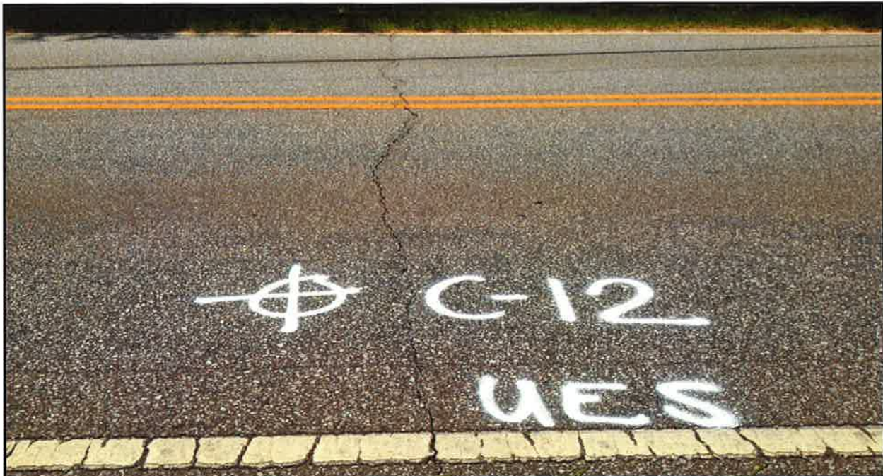
Photo 23: Transverse cracking, weathering and raveling.
