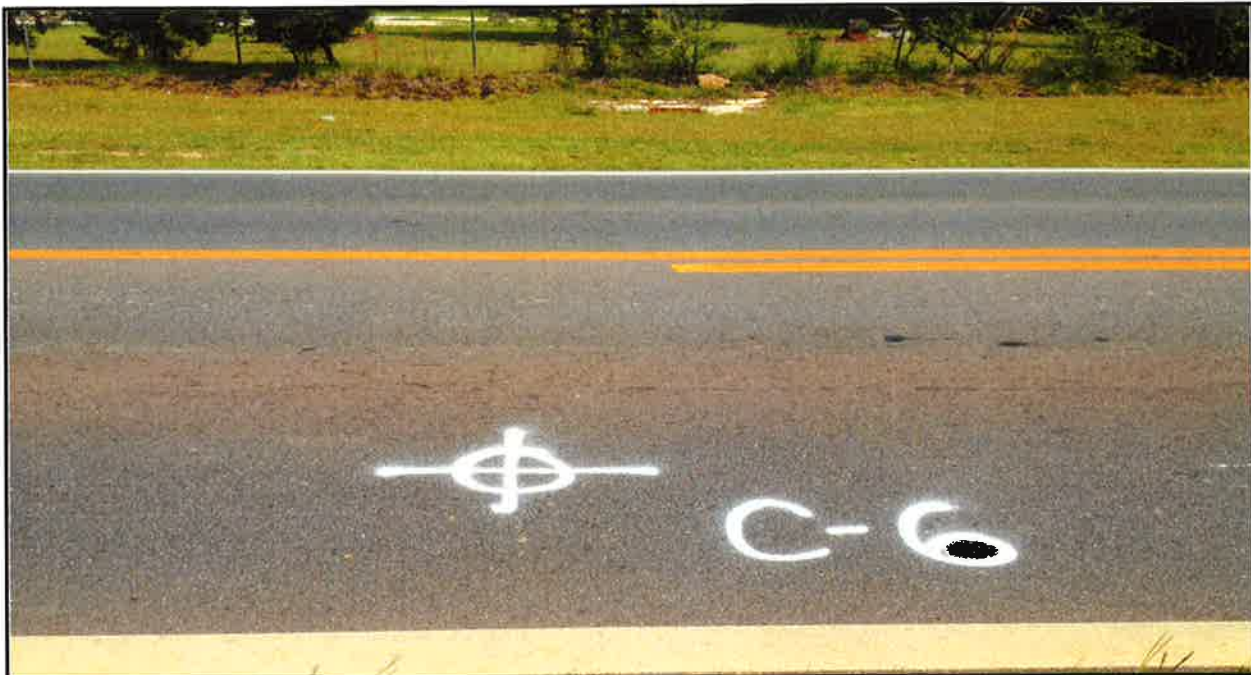
Photo 11: Pavement section looked good in the vicinity of core C-6 . Recently resurfaced.
