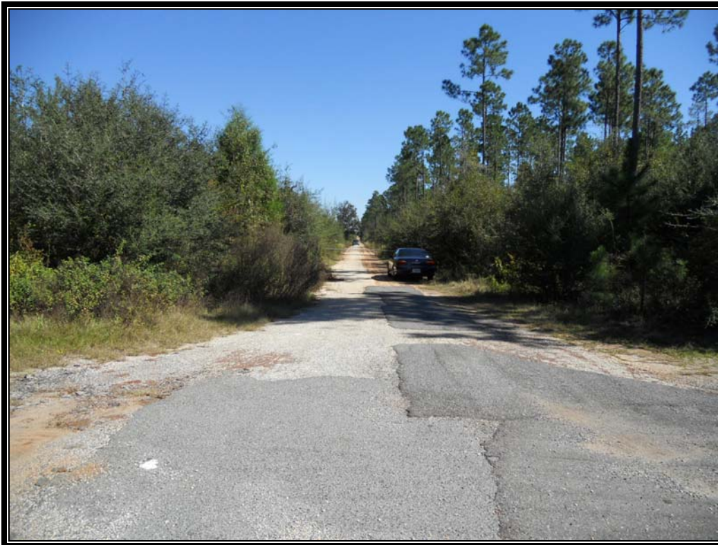
VIEW OF ACCESS ROAD TO - SUBJECT NOT SHOWN (SUBJECT PROPERTY IS ABOUT .5 MILES FROM ARD FIELD ROAD AND GATE)
