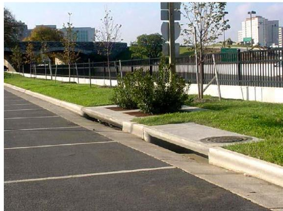
2. **Applicability** - Tree box filters can be used throughout Florida, and are especially useful in highly urbanized settings where available space is at a premium. They can be installed in open- or closed-bottomed chambers where infiltration is undesirable or not possible, such as clay soils, sites with high groundwater, and areas with highly contaminated runoff.
