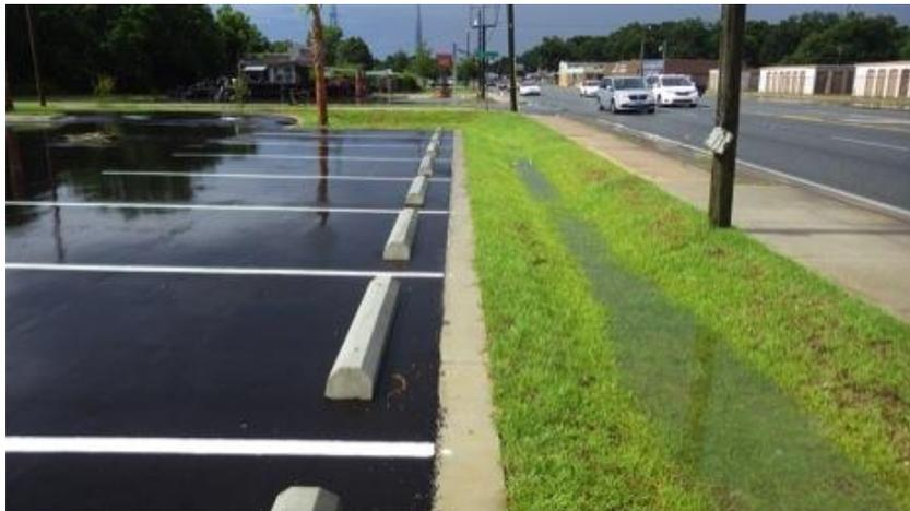
locations. Pavement must be graded so that stormwater flows through the curb cuts onto the vegetated area. Thus, roadways and other paved areas can be changed from DCIA to non-DCIA areas, reducing the calculated required treatment volume.
