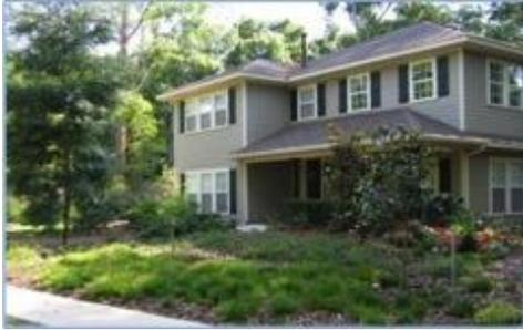
On sloping sites, rather than importing fill to make a level site for slab-on-grade foundations, use stem-wall construction and minimize the area disturbed and compacted. Fill material in Florida usually has a significantly different composition from native soils, particularly in the potential for phosphorus leaching.
