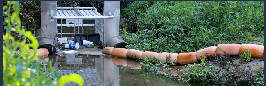
Floating litter trap at Jackson Creek in action
