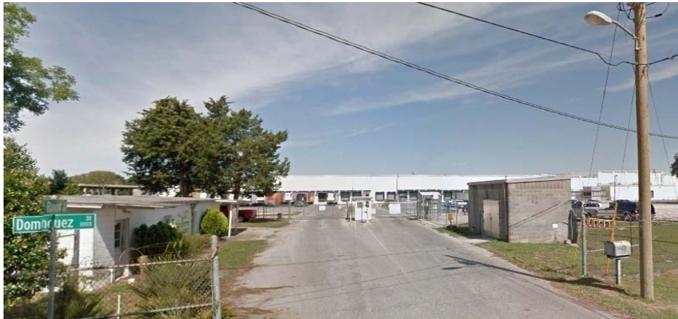
EXAMPLE OF A LIGHT INDUSTRIAL BUSINES ON DOMINIQUEZ AND BLOUNT STREET, PHOTO: GOOGLE MAPS
