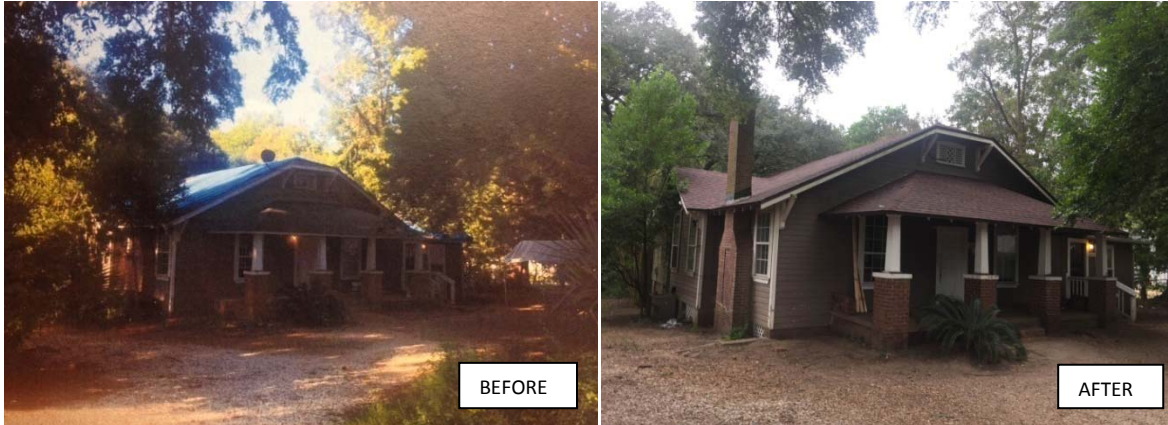
EXAMPLE OF A RESIDENTIAL REHABILITATION GRANT RECIPIENT, NEW ROOF INSTALLATION, PHOTO: CRA STAFF
