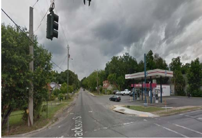
EXISTING CONDITION: WEST JACKSON STREET, GOOGLE MAPS
