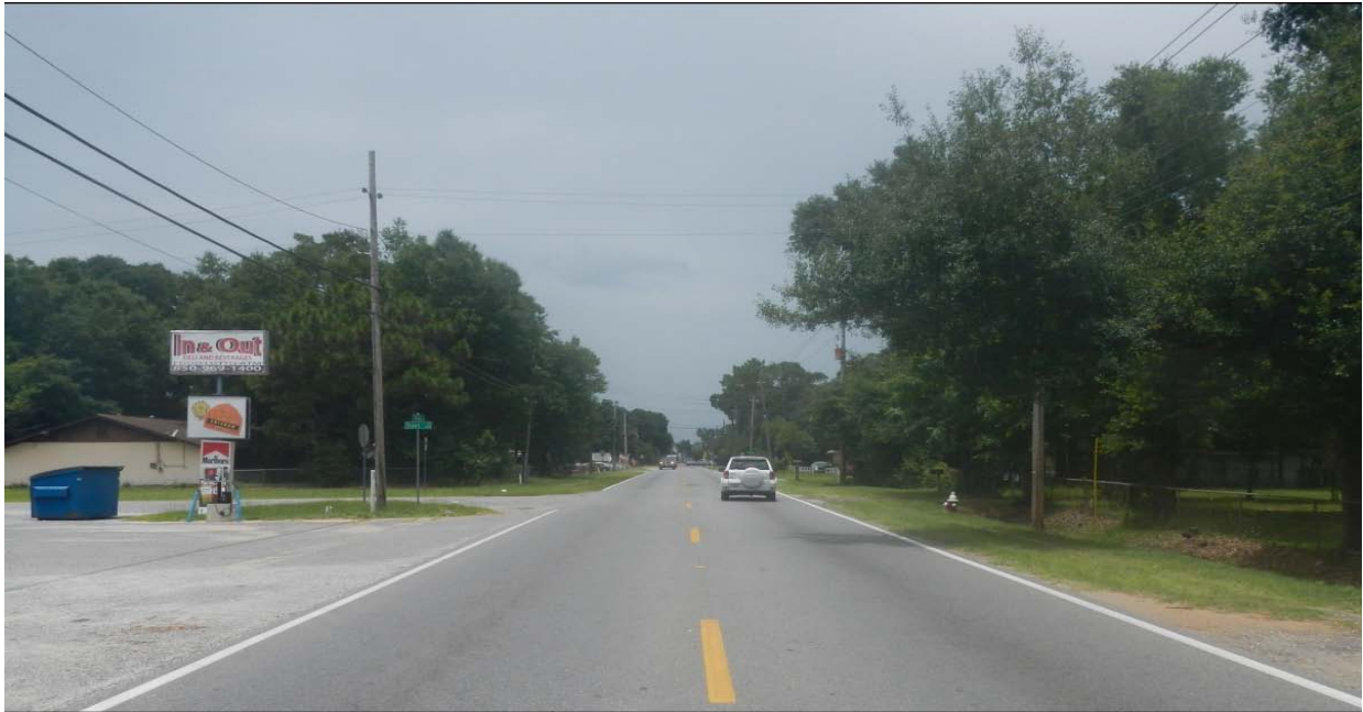
N. PALAFOX STREET CURRENT CONDITION, CREDIT: ATKINS GLOBAL, N. PALAFOX CORRIDOR MANAGEMENT PLAN, 2015
