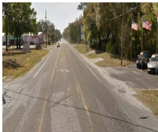
EXISTING CONDITION: E. OLIVE ROAD. CRA STAFF
