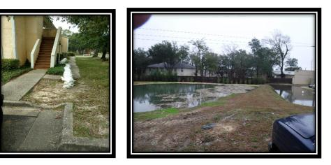
The Woodlands subdivision is located to the North of Nine Mile Rd. and has been impacted by several storm events. This project is to explore and design improvements to the existing drainage system to mitigate repeated flood conditions.
