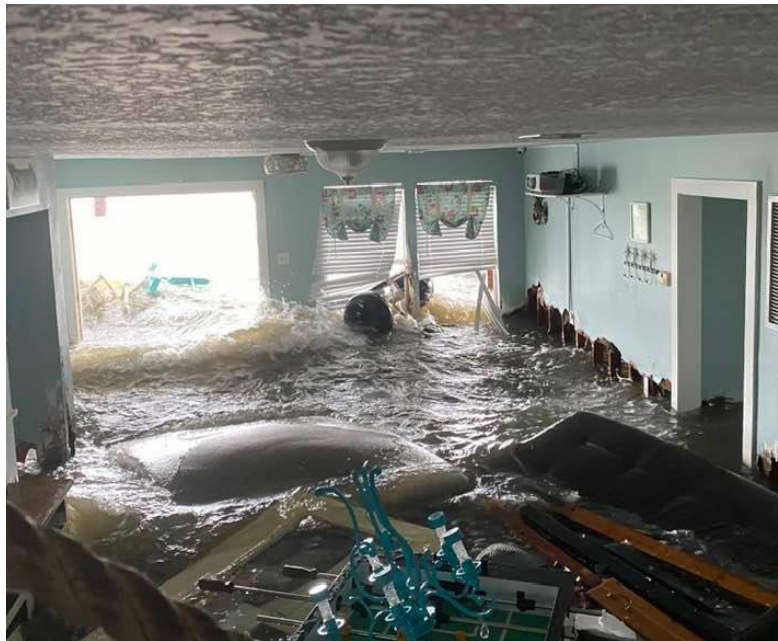
2020 flood damage - Hurricane Sally
