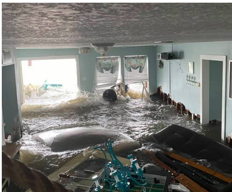
2020 flood damage - Hurricane Sally
