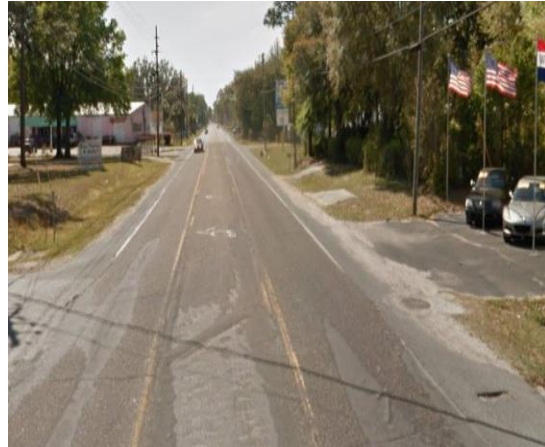
EXISTING CONDITION: E. OLIVE ROAD. CRA STAFF
