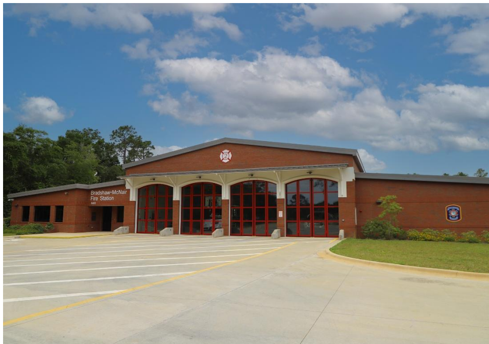
Figure 3: Beulah Fire Station
