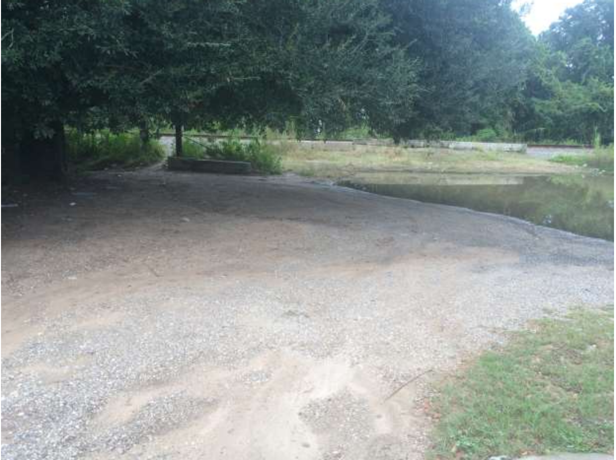
Flooding during 9/29/15 Flooding Event
