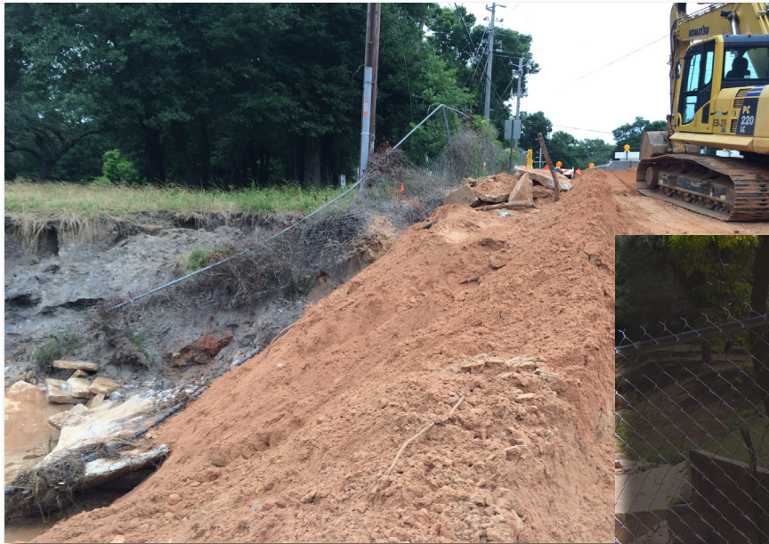
District 4 - East Johnson Avenue Culvert
