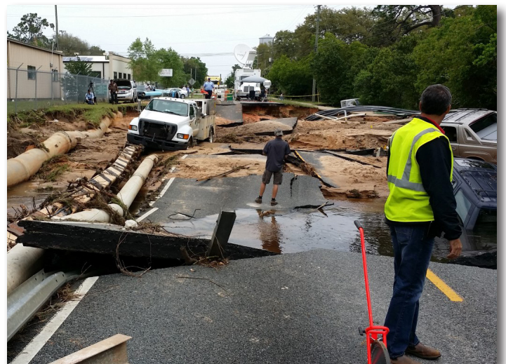
South Old Corry Field Road
