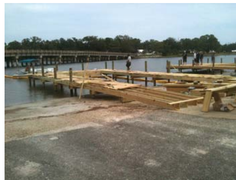
Figure 1: (Bottom & Top) Construction beginning at the boat ramp.
