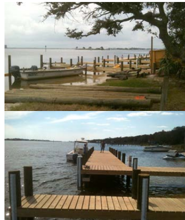
Figure 1: (Top) Construction of the boat ramp. (Bottom) Completion of the ramp.
