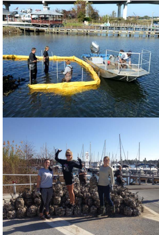
Figure 3: (Bottom & Top) Volunteers and State workers construct the oyster reef.
