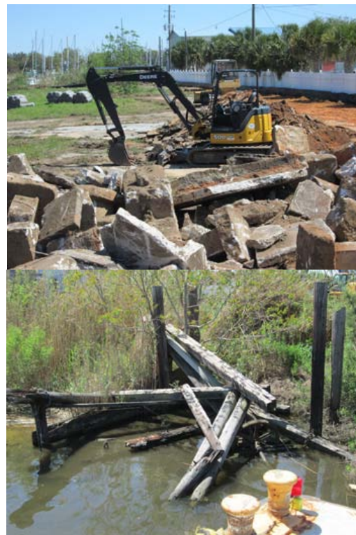
Figure 1: (Bottom & Top) Construction beginning at the boat ramp.
