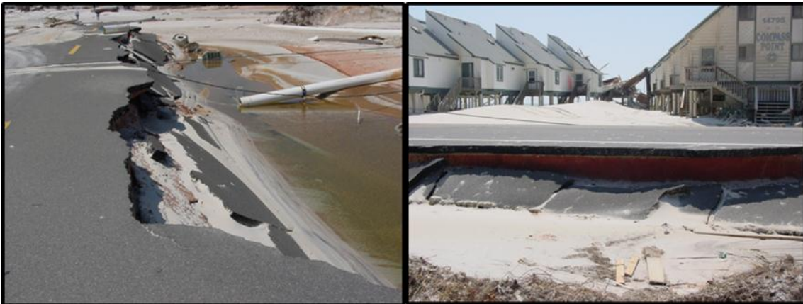
Figure 10. Hurricane damage to SR 292 and nearby habitat for the PKBM in 2004.
