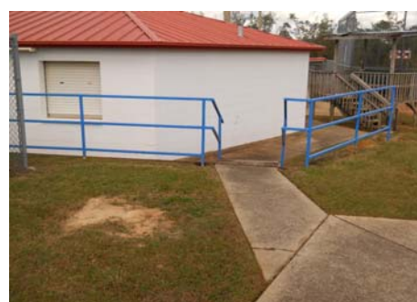
Building 6 Restrooms & Concession
