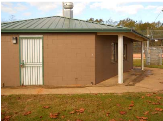
Building 3 Restrooms & Concession
